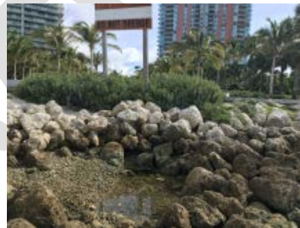
Figure 5: Rip-rap energy dissipation near outfall
