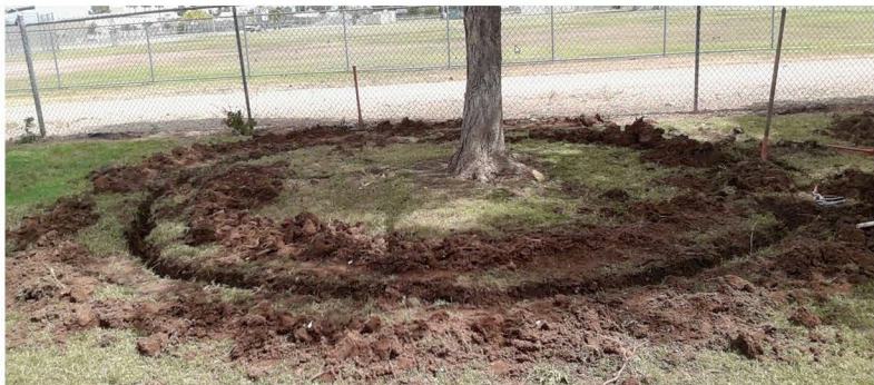
Trench Opened to Access Roots
