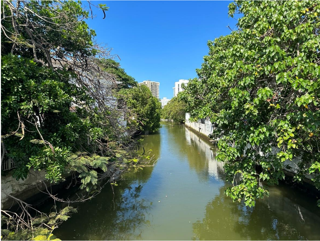
Collins Canal at 23 rd Street (looking east)
