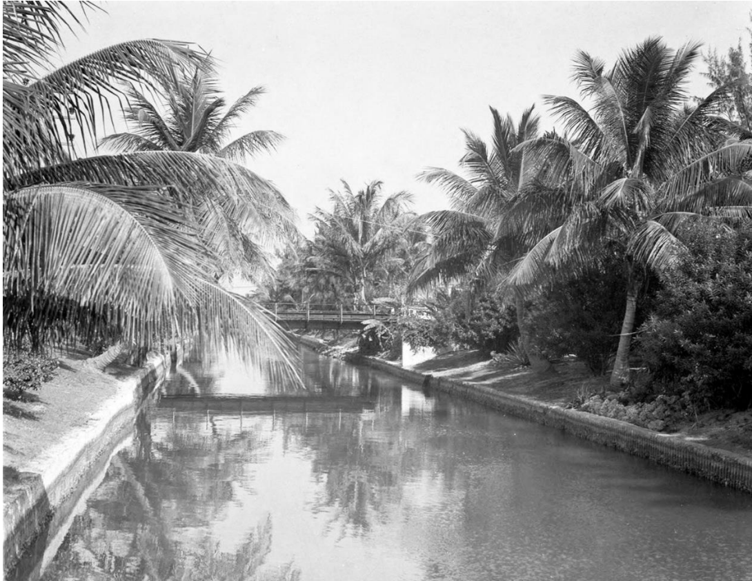
Close up of Collins Canal, 1931
