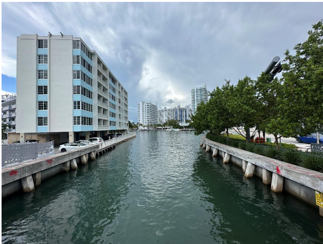
Collins Canal at Lincoln Court Pedestrian Bridge (looking west)
