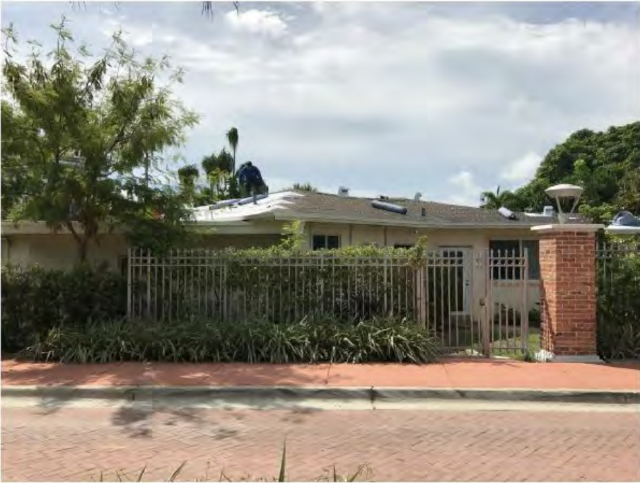
2 7678 BAYSIDE LANE (EAST ALONG BRIDGE) 2016/09/24
