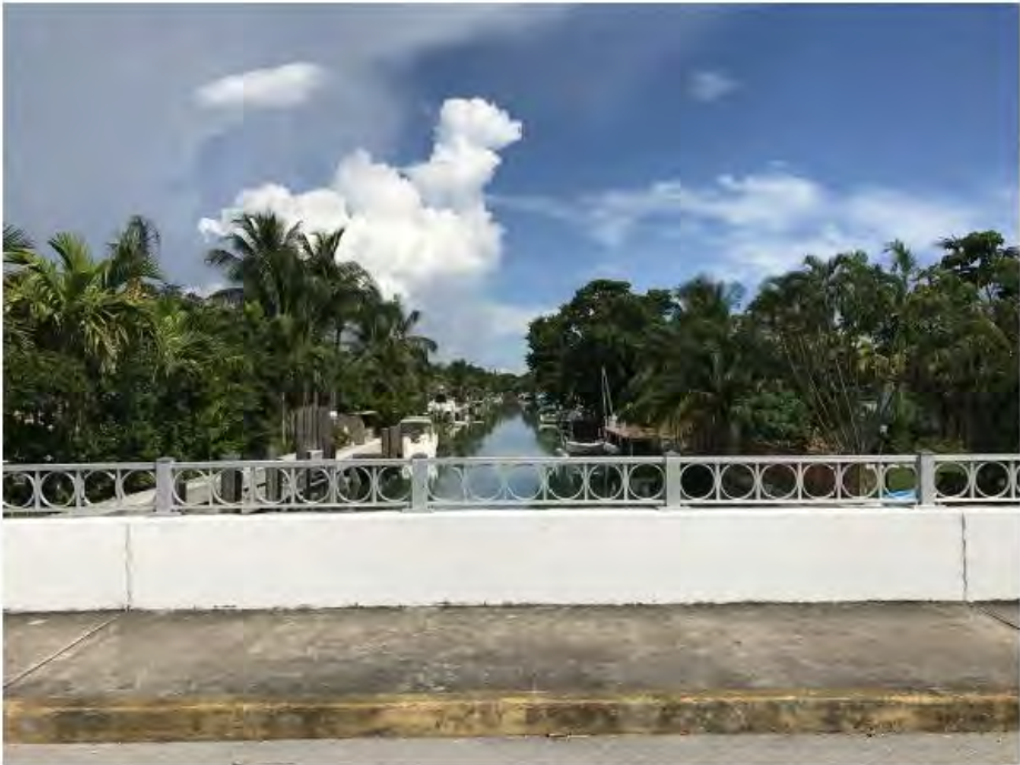
53 S, BISCAYNE POINT RD BRIDGE (LOOKING EAST) 2016/09/24
