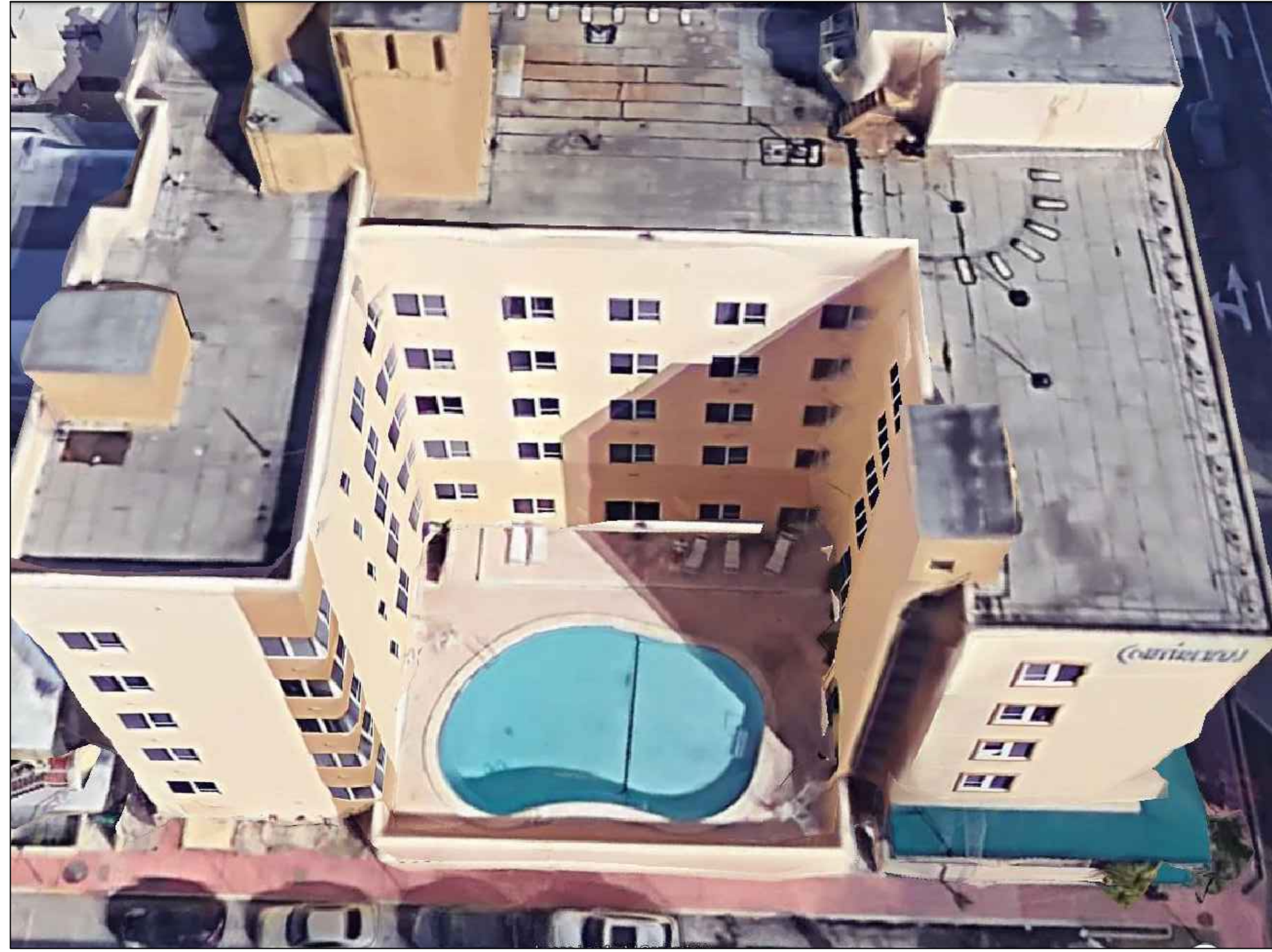
VIEW 1 EXIST. POOL – CONTINENTAL HOTEL – AERIAL VIEW
