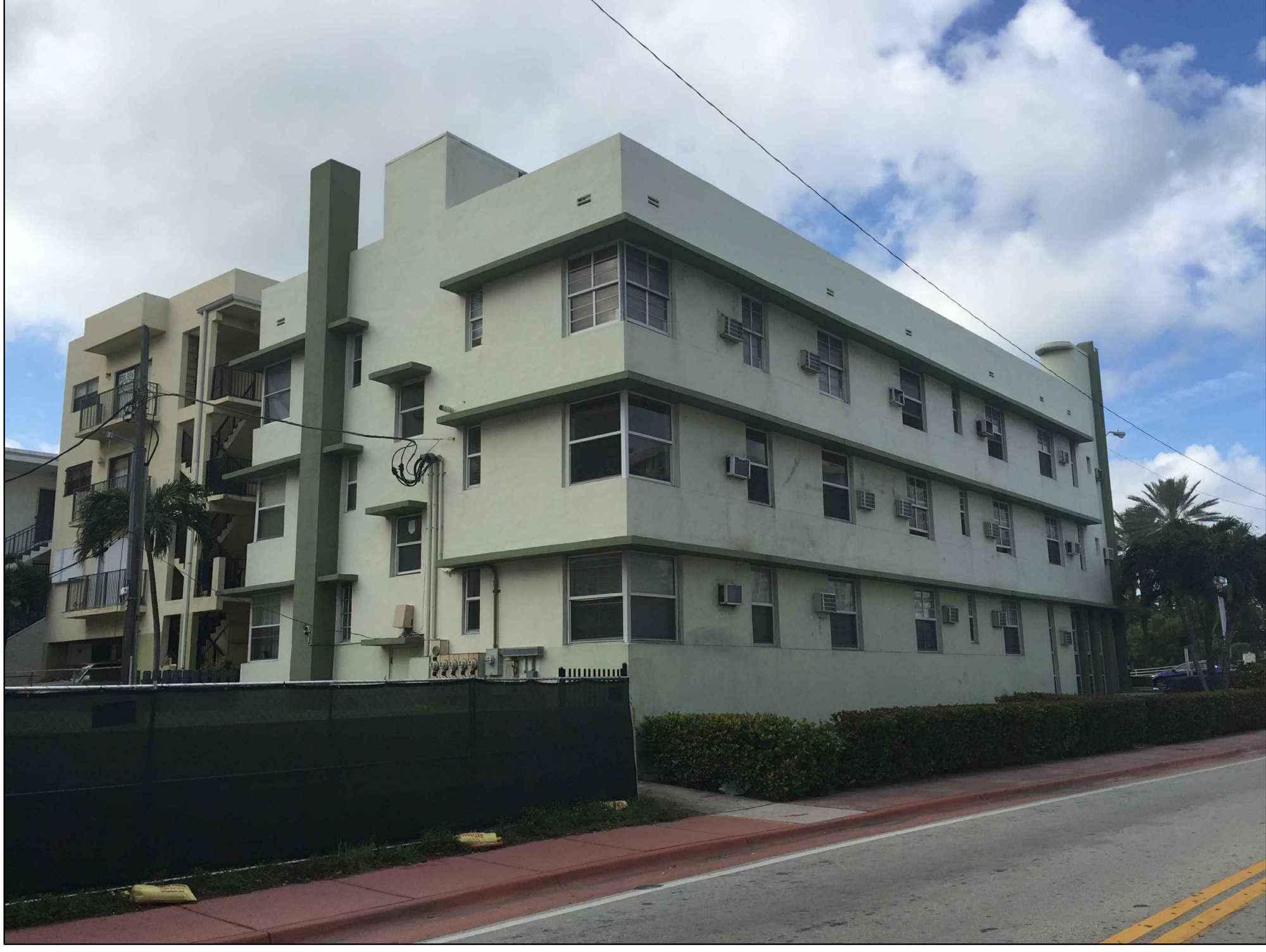
VIEW 2 RESIDENTIAL BUILDING
