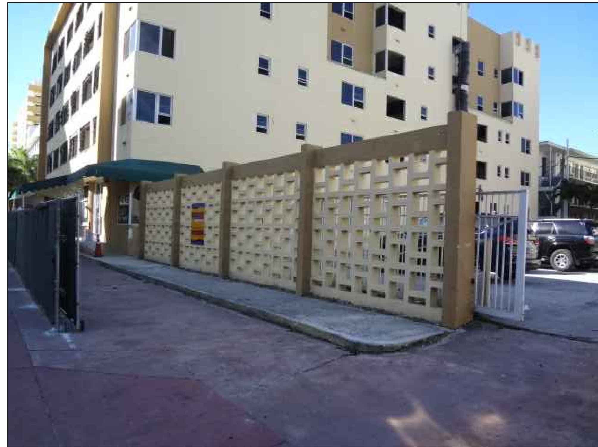
VIEW 4 DECORATIVE WALL TO BE DEMOLISHED @ SOUTH WEST CORNER OF THE BUILDING
