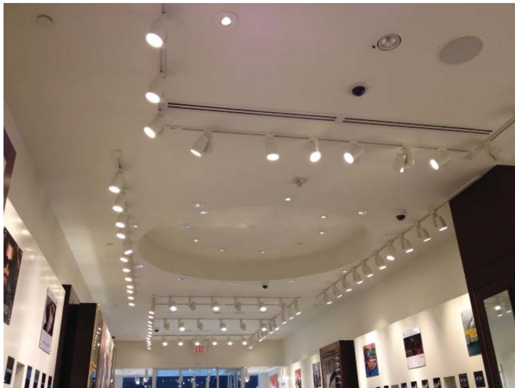
Dropped ceiling in 805 Lincoln Road, possibly obscuring historic wood ceiling
