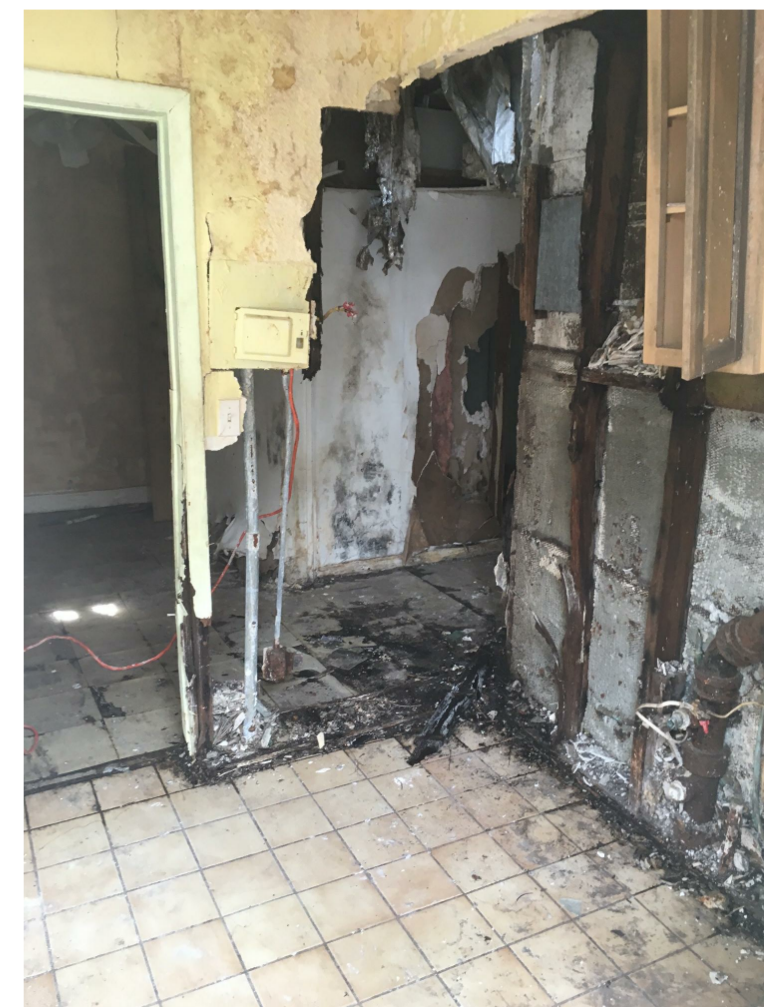
EXISTING BUILDING INTERIOR VIEW AT BATHROOM
