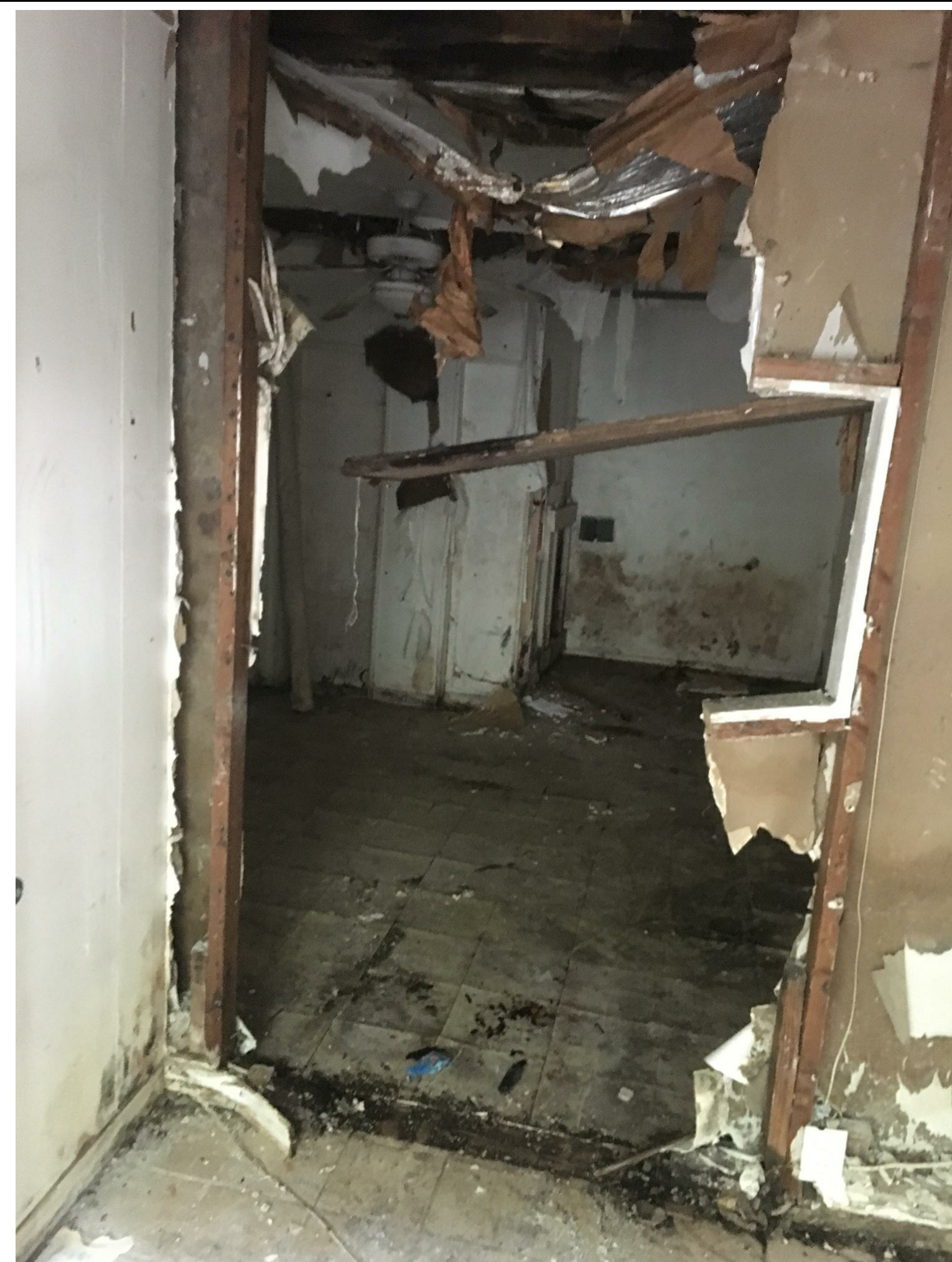
EXISTING BUILDING INTERIOR VIEW AT BEDROOM
