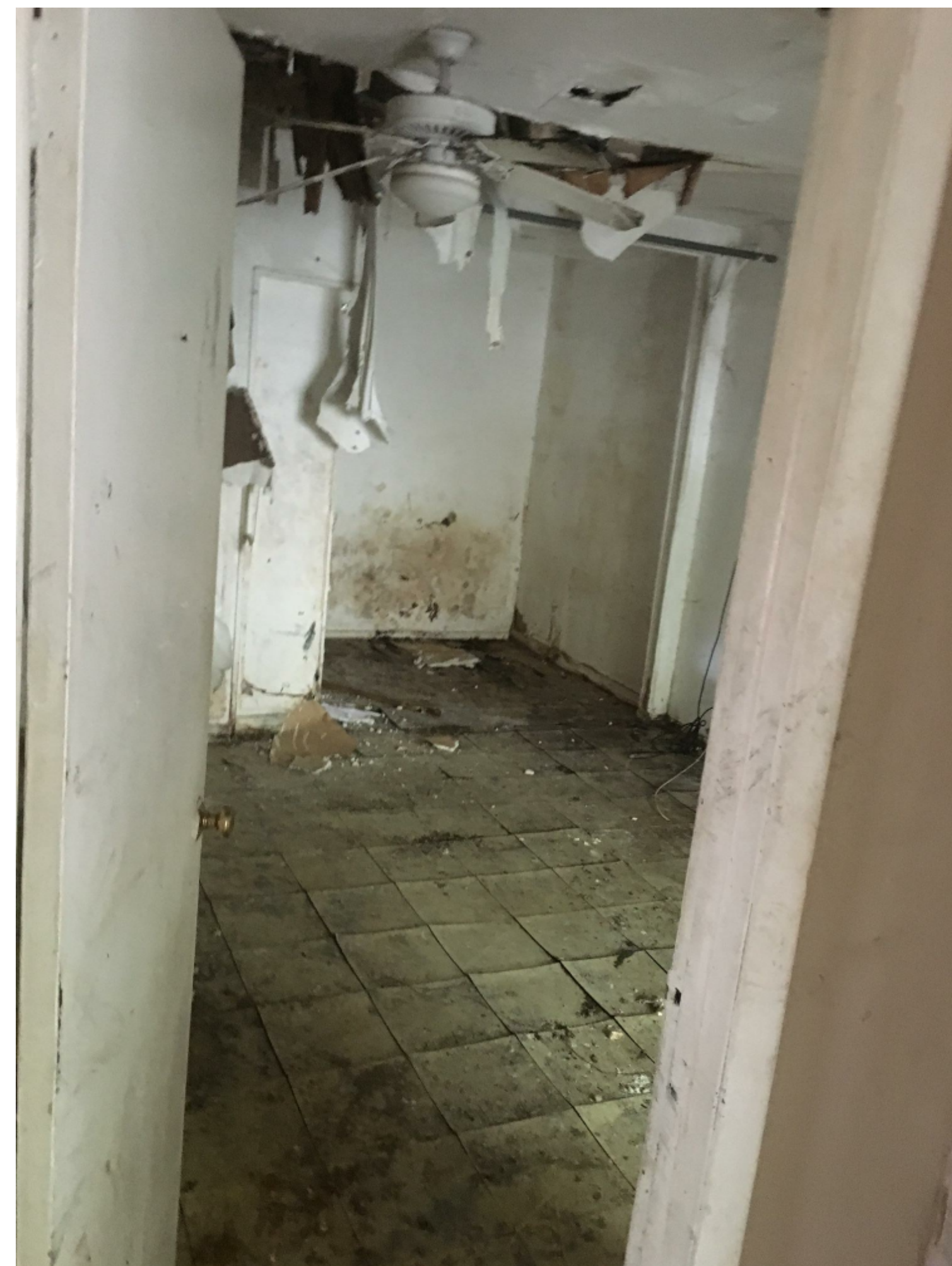
EXISTING BUILDING INTERIOR VIEW AT BEDROOM
