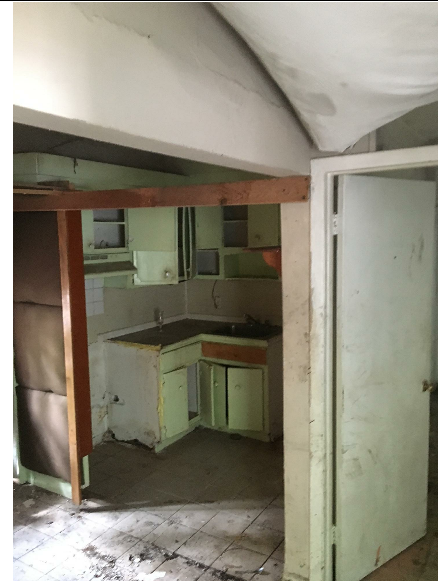
EXISTING BUILDING INTERIOR VIEW AT KITCHEN
