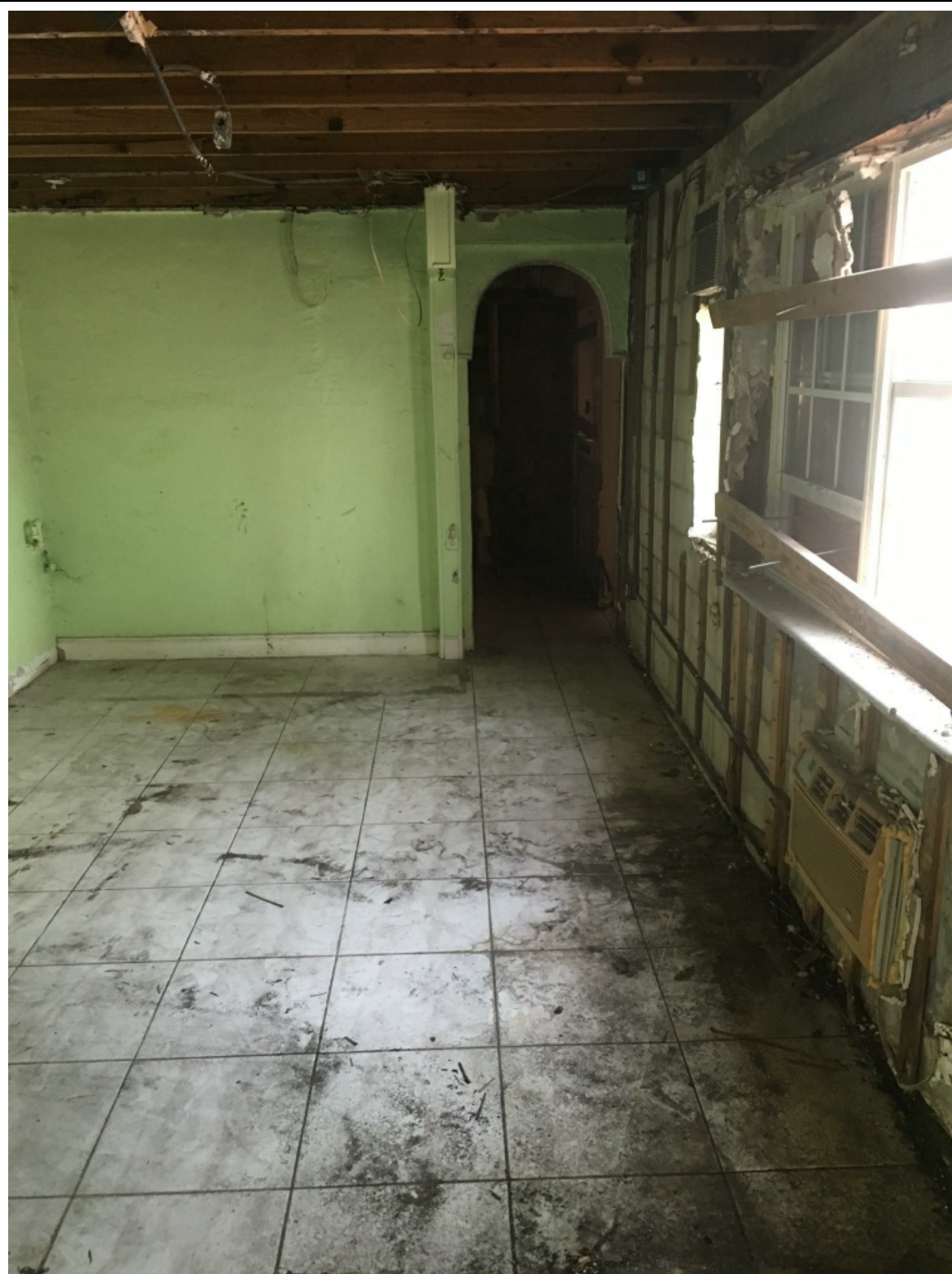
EXISTING BUILDING INTERIOR VIEW AT LIVING ROOM
