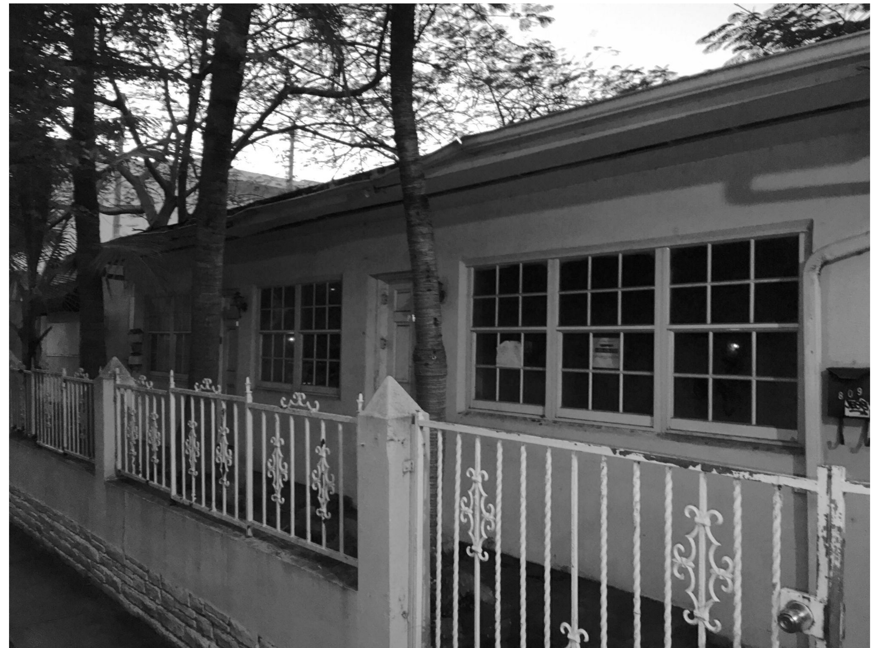
809 2ND ST. SOUTH ELEVATION (FROM EAST)
