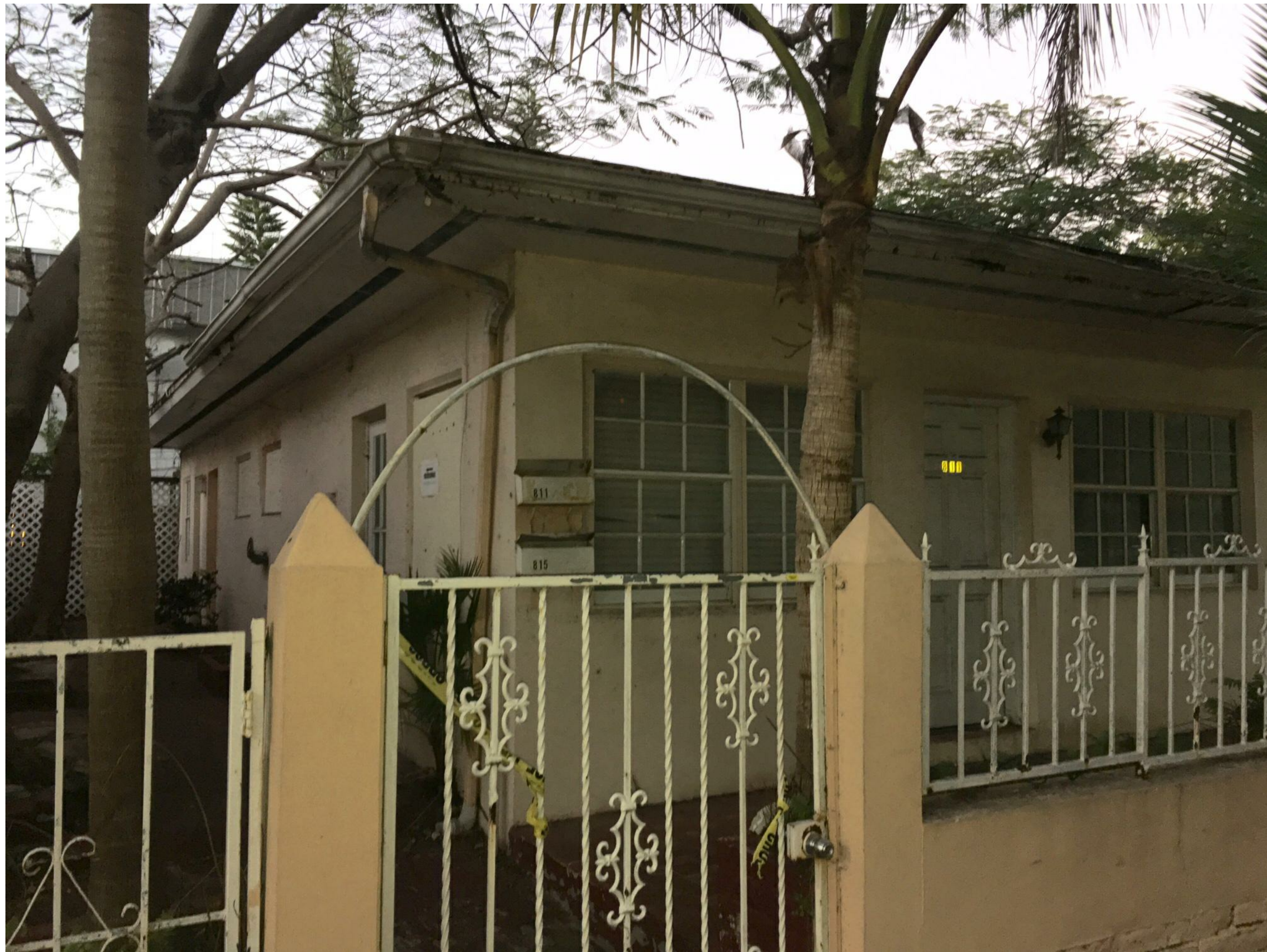
809 2ND ST. SOUTH-WEST CORNER
