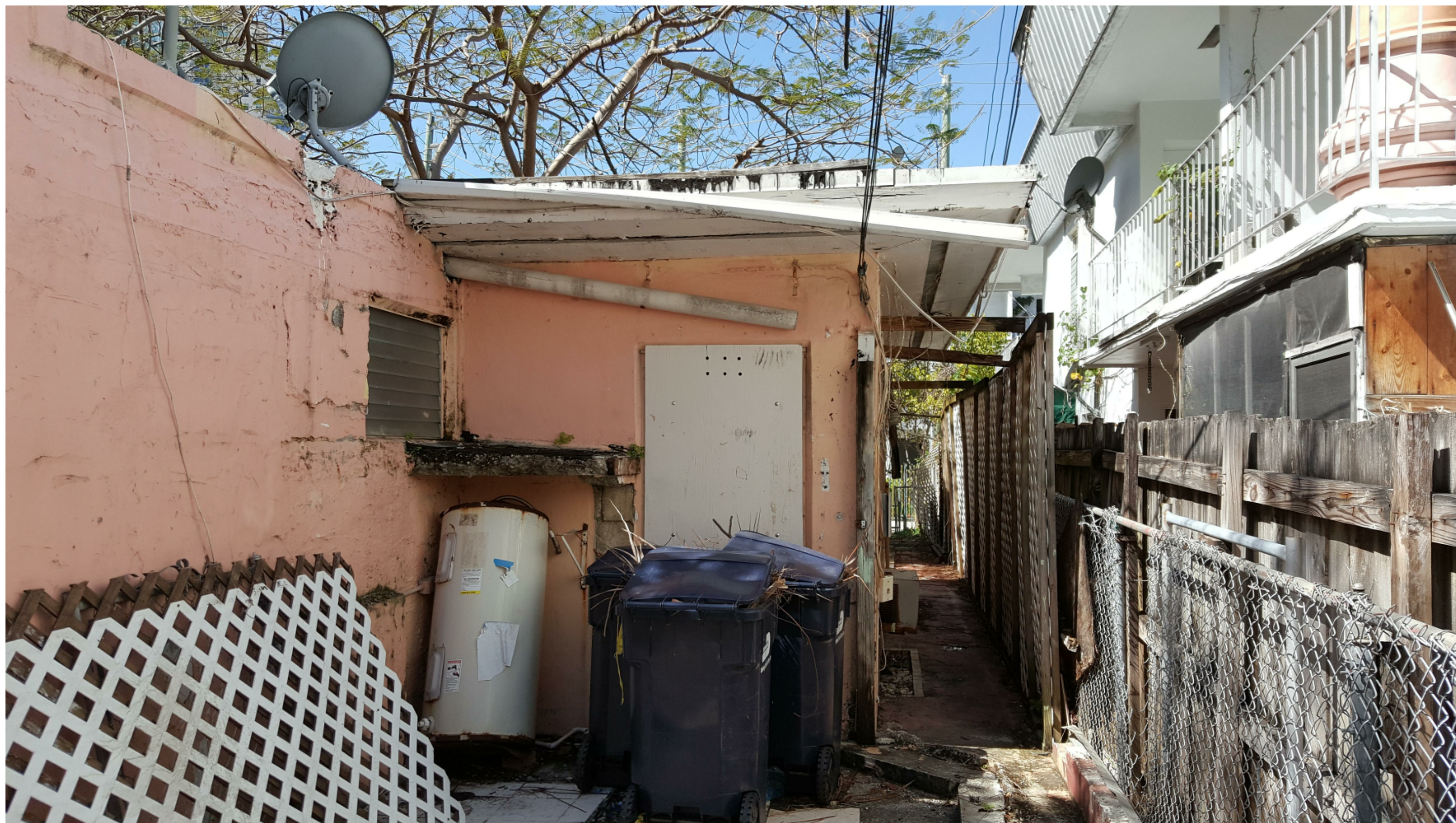
809 2ND ST. EAST ELEVATION (NORTH END)
