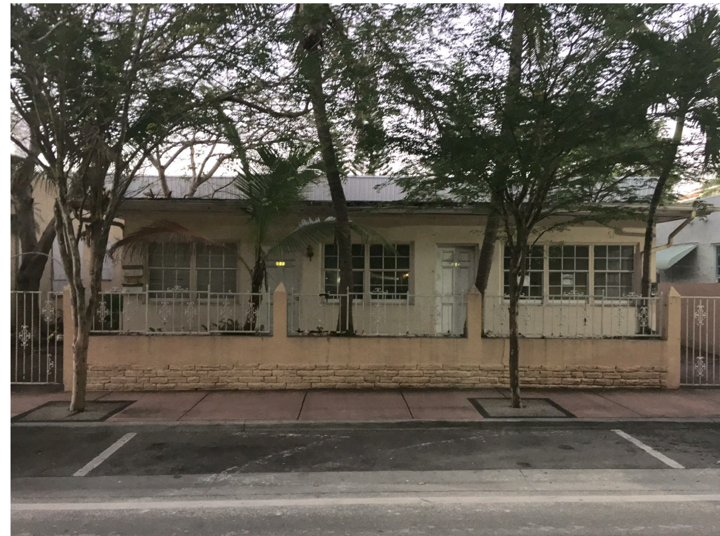
809 2ND ST. SOUTH FACADE
