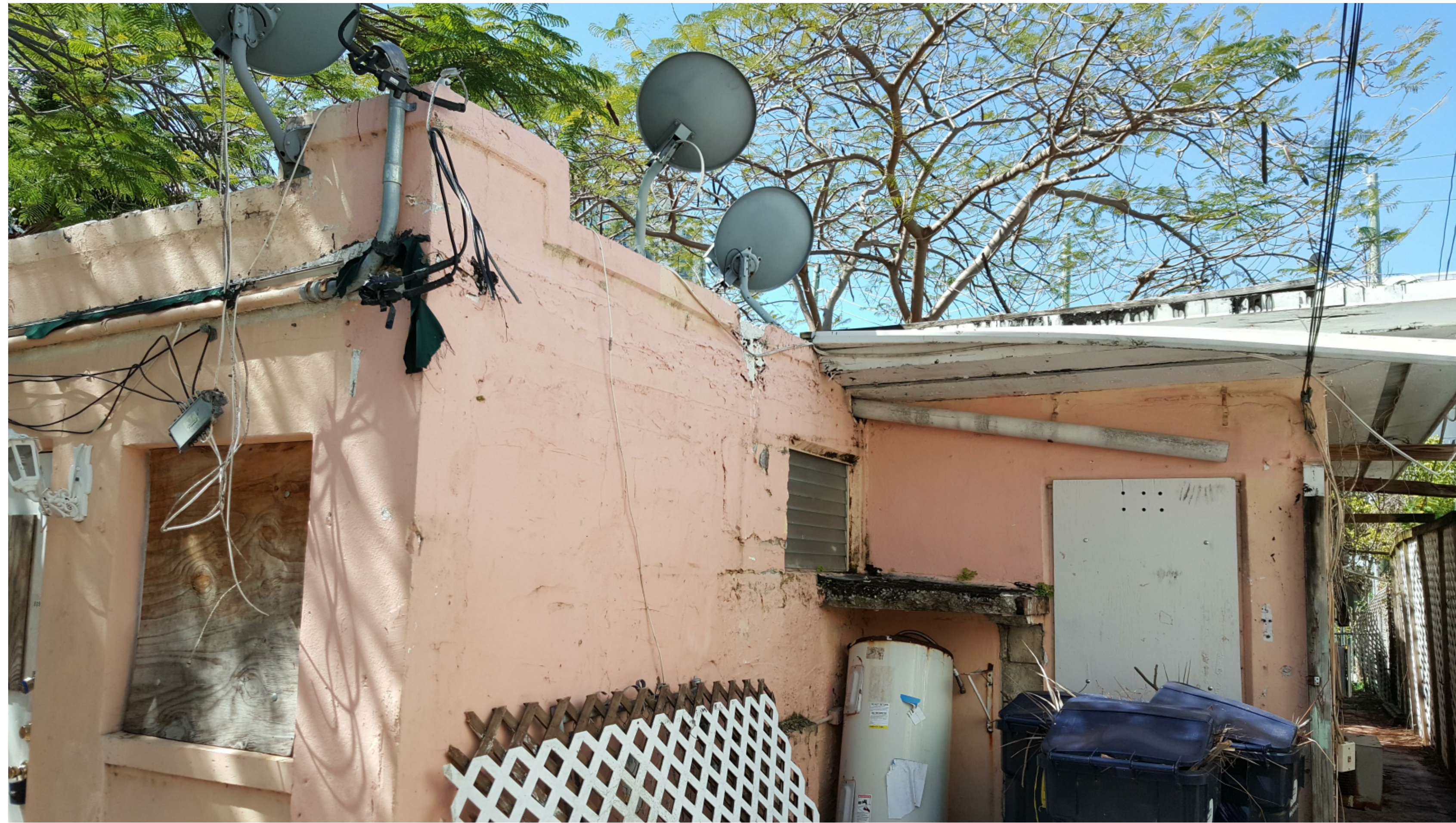
809 2ND ST. EAST ELEVATION (FROM NORTH)
