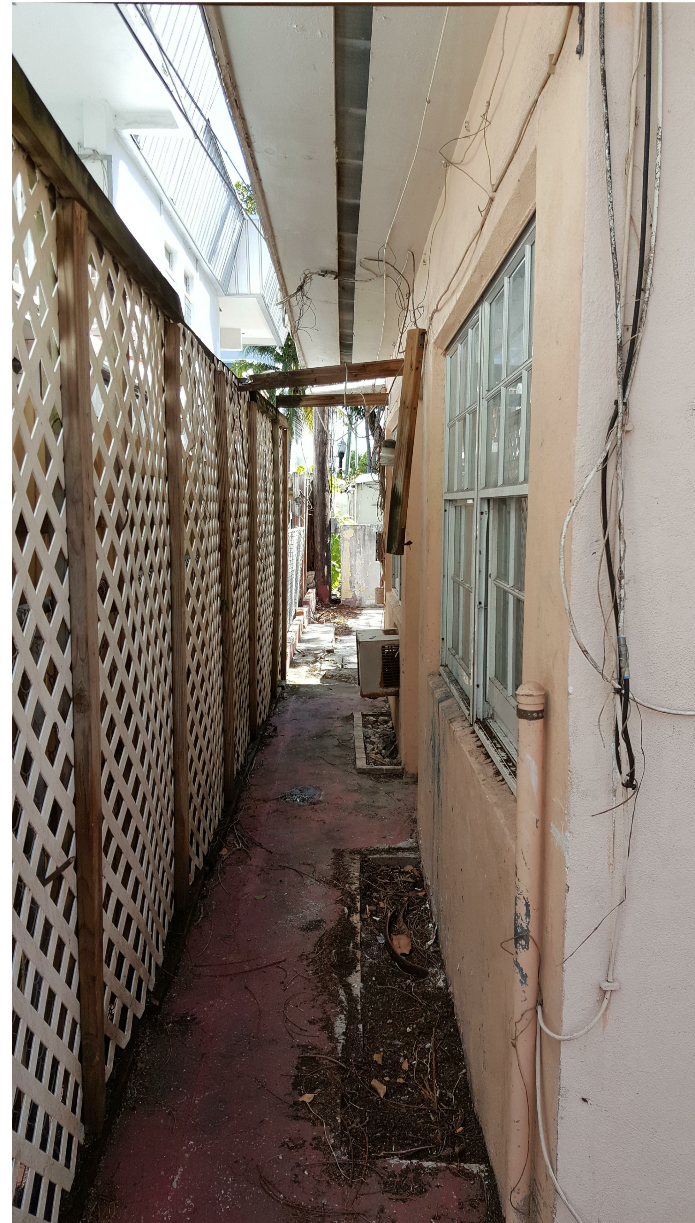
809 2ND ST. NORTH ELEVATION (REAR)
