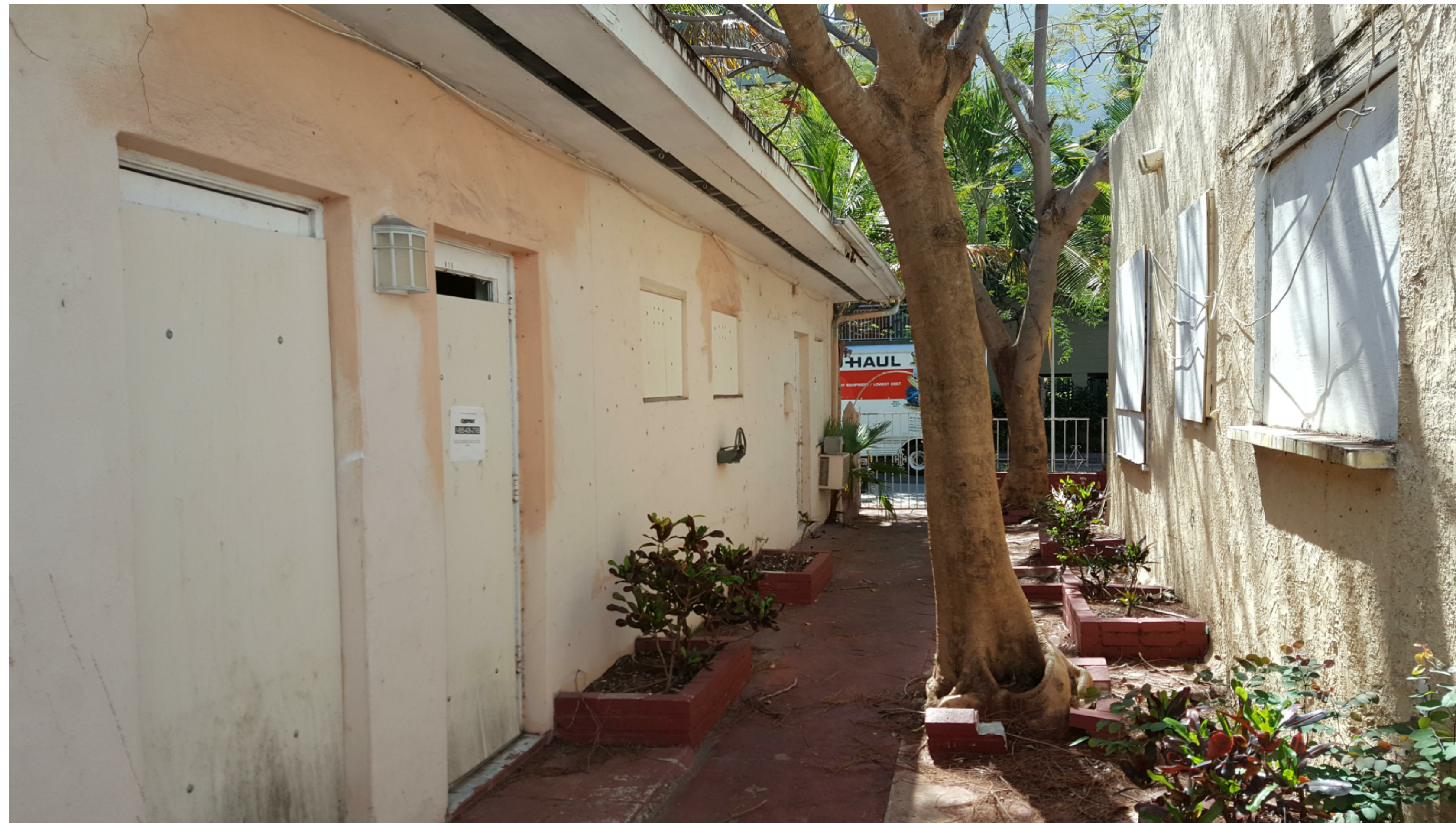
809 2ND ST. WEST ELEVATION (FROM NORTH)
