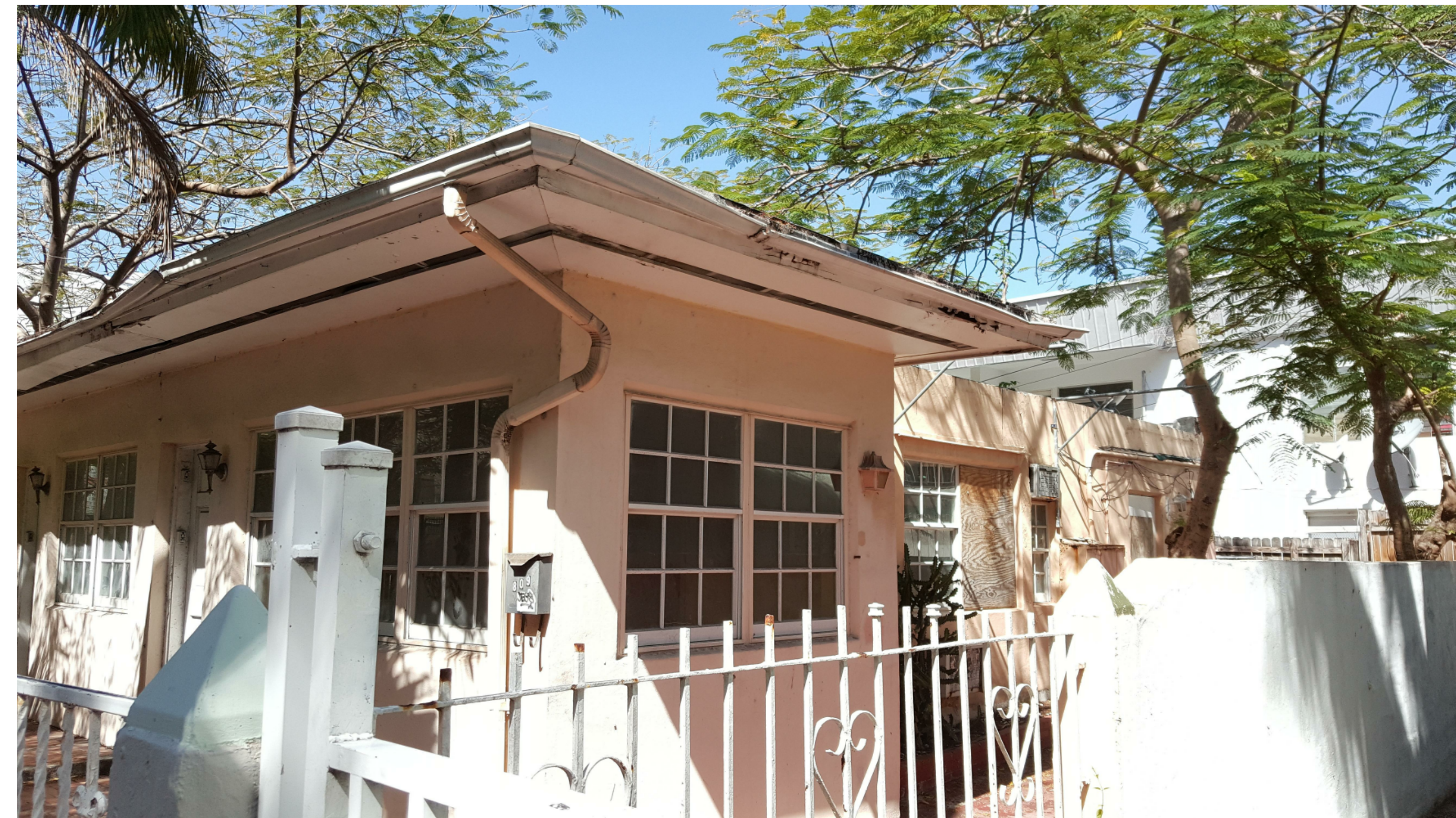
809 2ND ST. EAST ELEVATION (FROM SOUTH)
