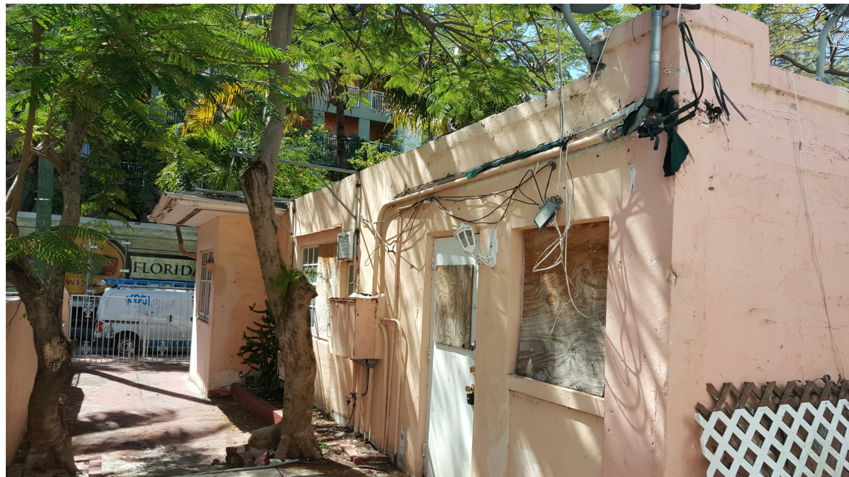
809 2ND ST. EAST ELEVATION (FROM NORTH)
