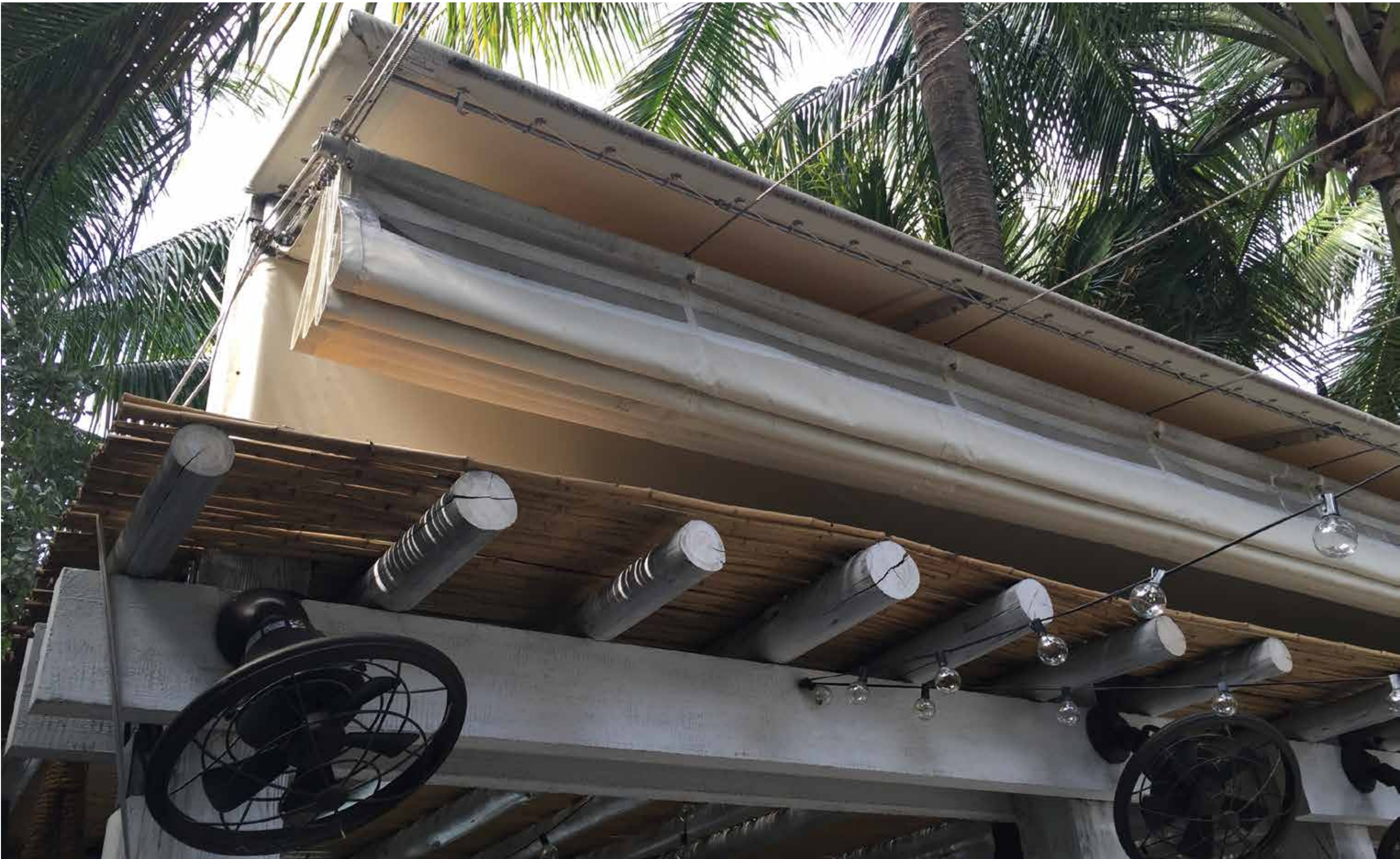
P-39: EXISTING OPEN SPACE SITE CONDITION (retractable awning detail)
