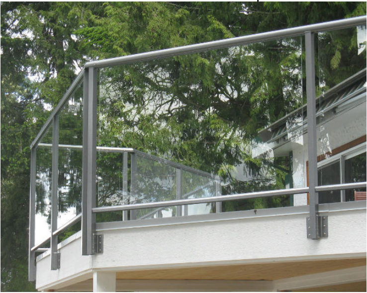
Glass Railing with Aluminum Posts
