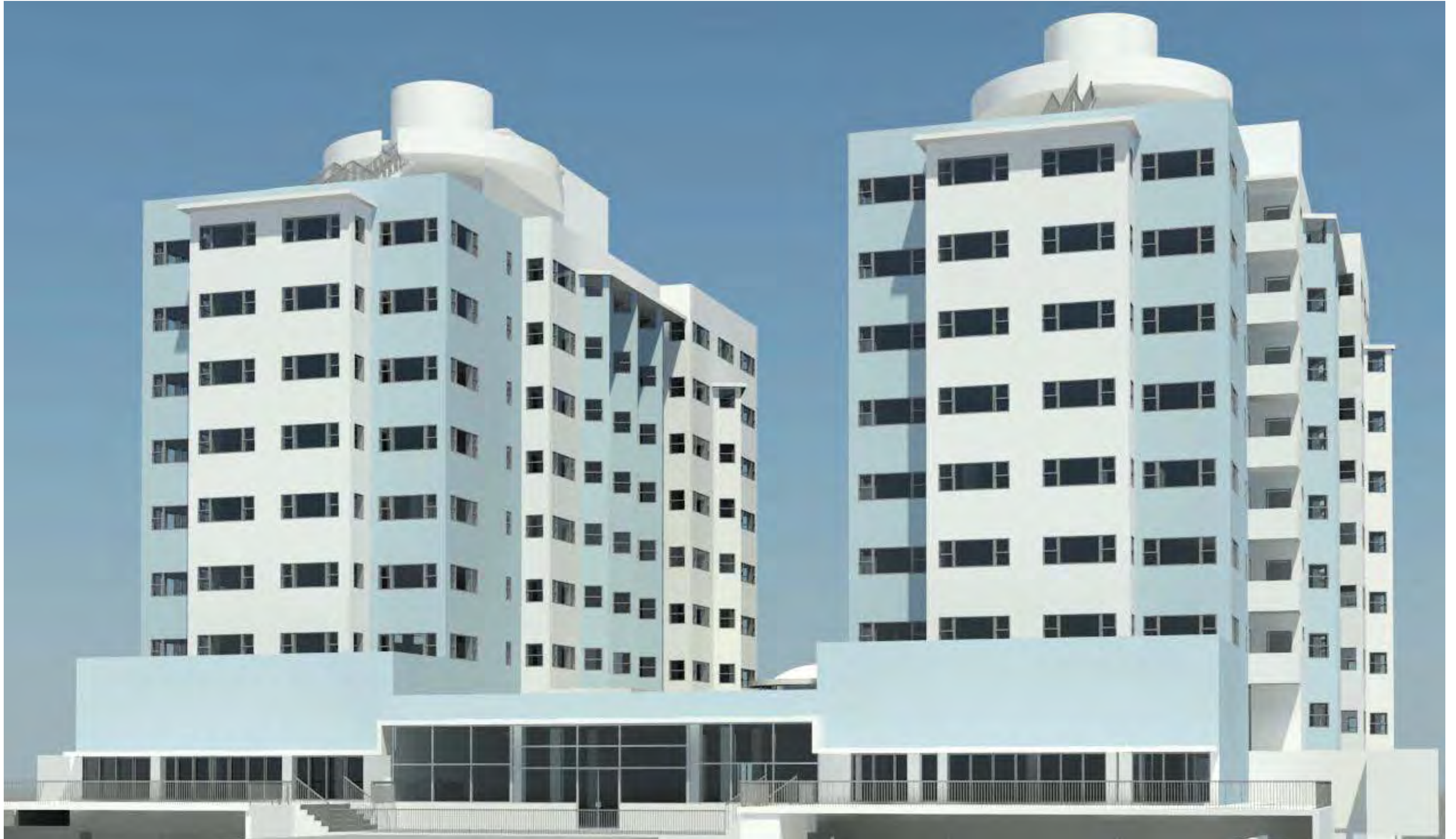
OCEAN FRONT VIEW FROM EAST / EXISTING 12-14-2015
