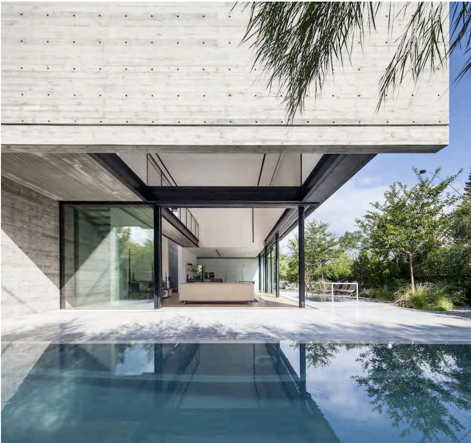
SLIDING DOORS & OFF-FORM CONCRETE WALLS
