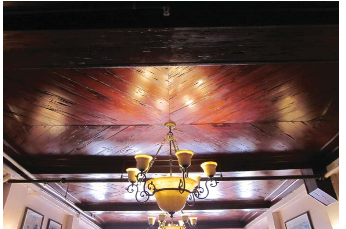
⑤ EXISTING CEILING(PRESENT)
