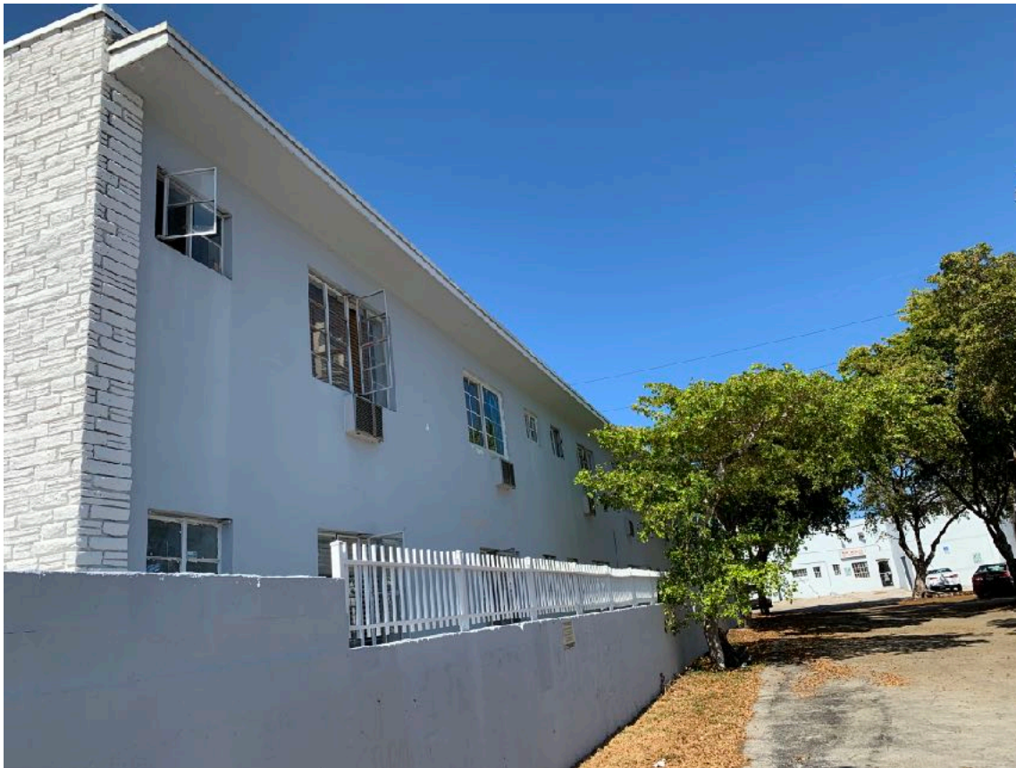
7435 HARDING AVENUE EXISTING CONDITION
