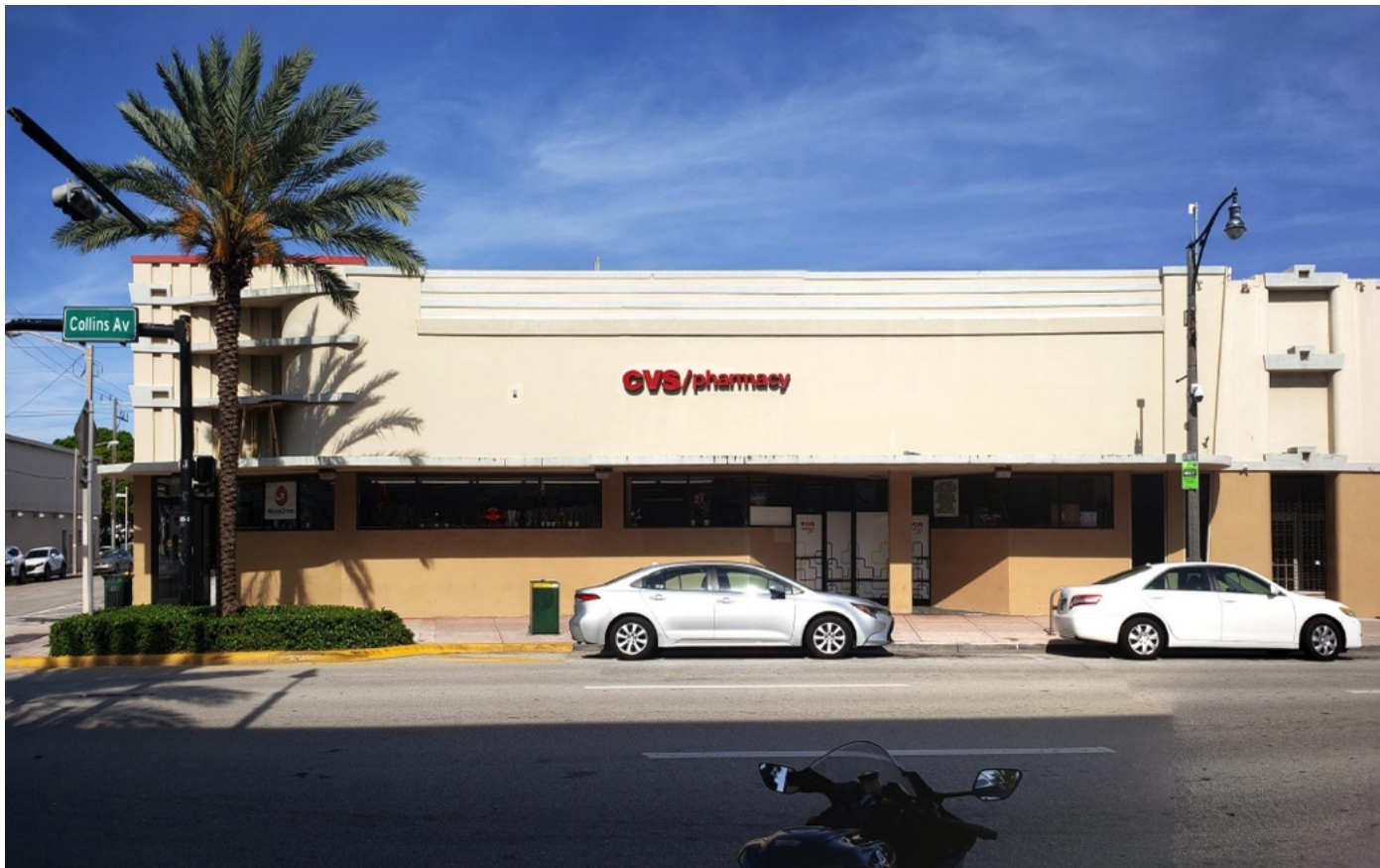
14. COLLINS AVE - EXISTING CVS
