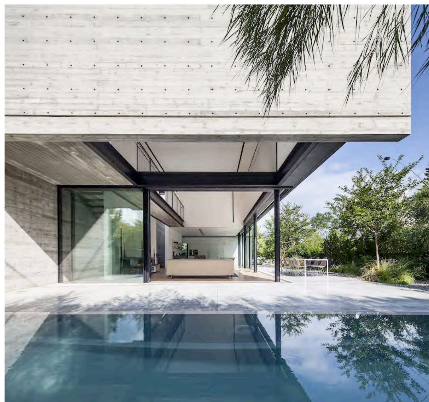
SLIDING DOORS & OFF-FORM CONCRETE WALLS
