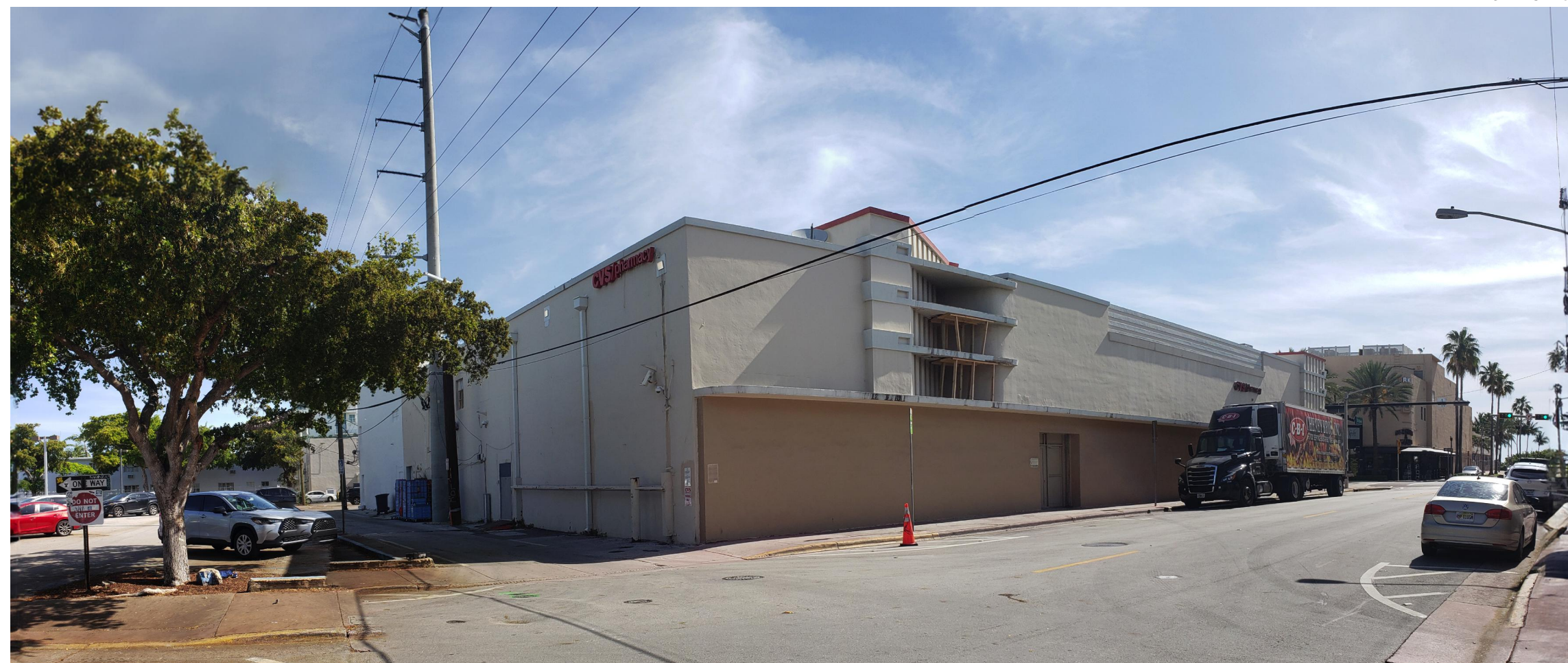
10. Alley entrance from 74th Street
