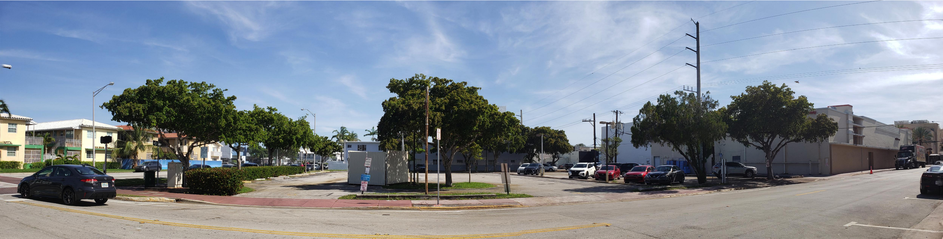
9. View towards Harding site from 74th street
