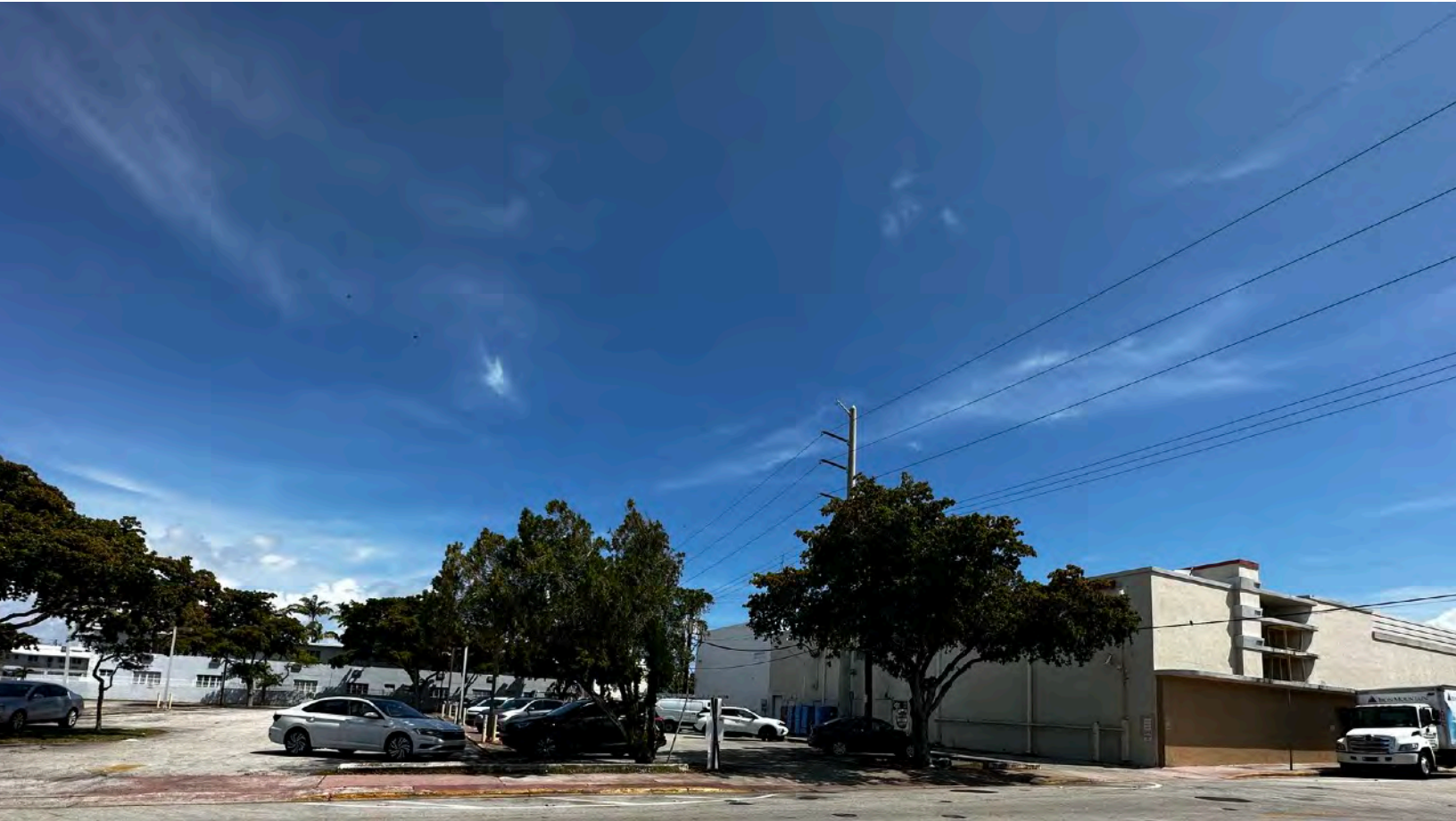
WEST ELEVATION WITH REAR PARKING LOT (11)
