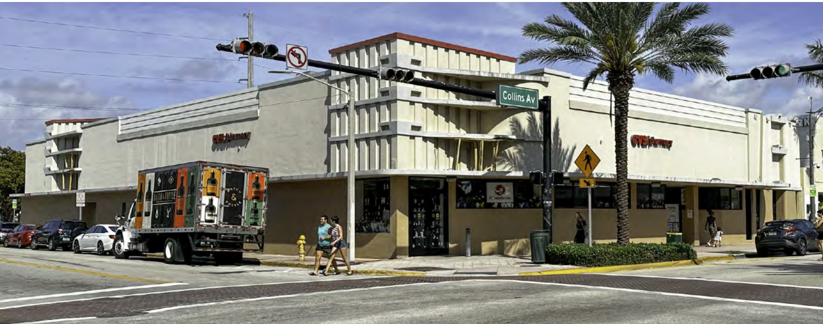
2023 PHOTOGRAPH of NW CORNER OF 74th & COLLINS AVENUE WITH EAST AND SOUTH ELEVATIONS
