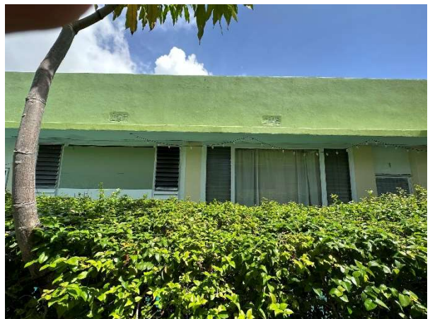
Figure 102. View of Unit 11, looking north, August 2023.
