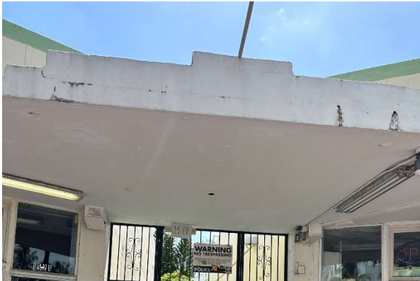
Figure 74. Detail of ziggurat over entrance to walkway, August, 2023.
