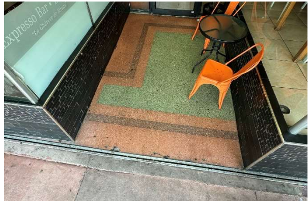
Figure 57. Detail of partially obscured terrazzo at entrance to 1499 Washington Avenue, August 2023.
