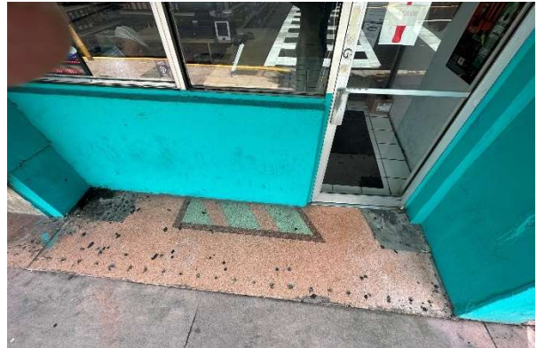
Figure 51. Detail of partially obscured terrazzo at entrance to 1491 Washington Avenue, August 2023.
