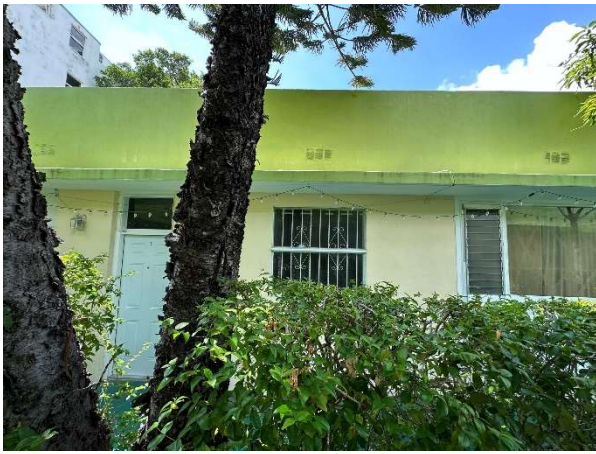
Figure 97. View of Unit 5, looking south, August 2023.
