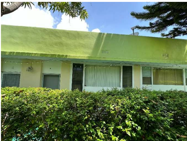
Figure 101. View of Unit 10, looking north, August 2023.
