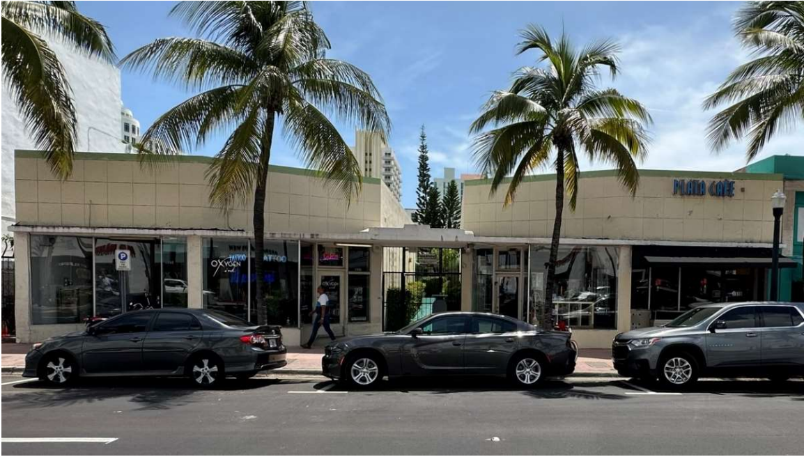
Figure 2. 1515-1523 Washington Avenue, August 2023.
