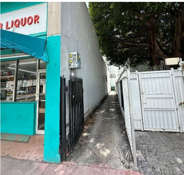
Figure 36. View of alley along south elevation, looking east, August 2023.
