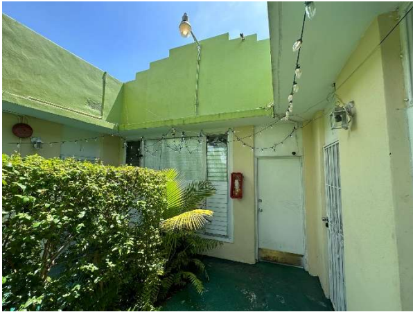
Figure 99. View of Unit 7, looking east, August 2023.
