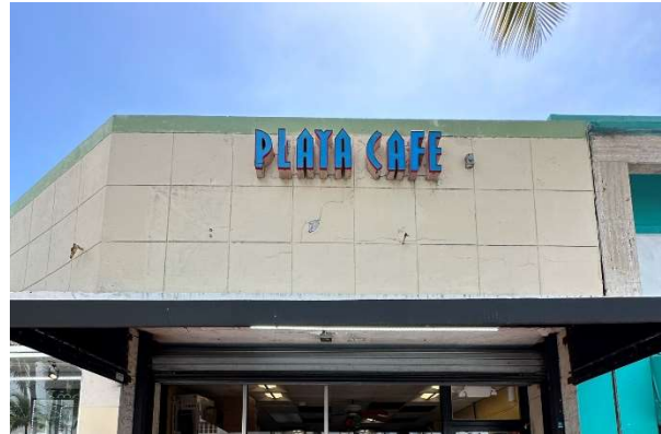
Figure 75. Detail of square concrete panels above canopy, August, 2023.
