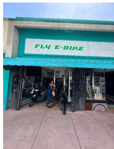
Figure 49. View of 1513 Washington Avenue, August 2023.
