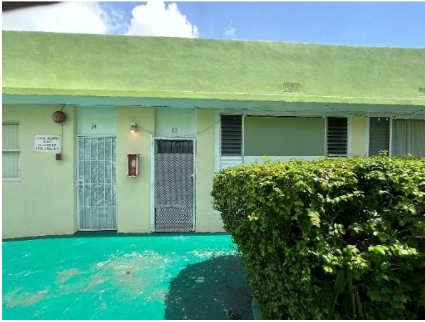
Figure 103. View of Unit 12, looking north, August 2023.
