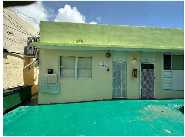
Figure 104. View of Unit 14, looking north, August 2023.
