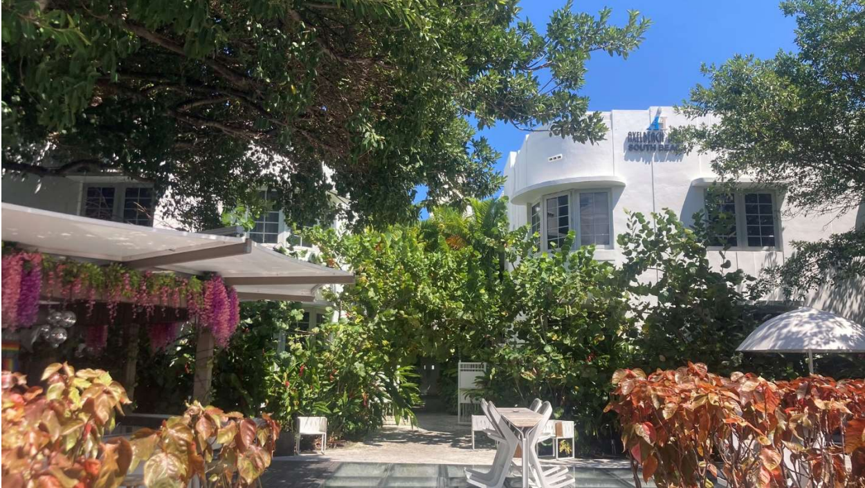
Figure 2. 1453-55 Washington Avenue, September 2023.
