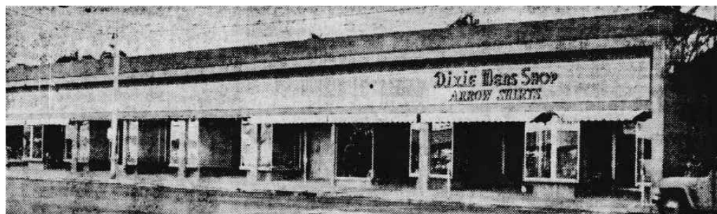
AT MIAMI BEACH, this new commercial building, containing nine store units, has just been completed at 15th st. and Washington ave. for Daniel I. Taradash. Constructed by the Leifer Construction Co. from plans drawn by Architect Albert Anis, the building fronts 140 feet on Washington ave. and extends 80 feet in depth. Management of the building is by Taradash Properties, 927 Lincoln rd.
