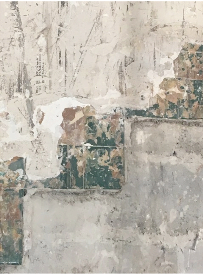
LEFT PHOTO: DETAIL SHOWING ORIGINAL GLAZED TILE FORMING STAIR BASEBOARD
