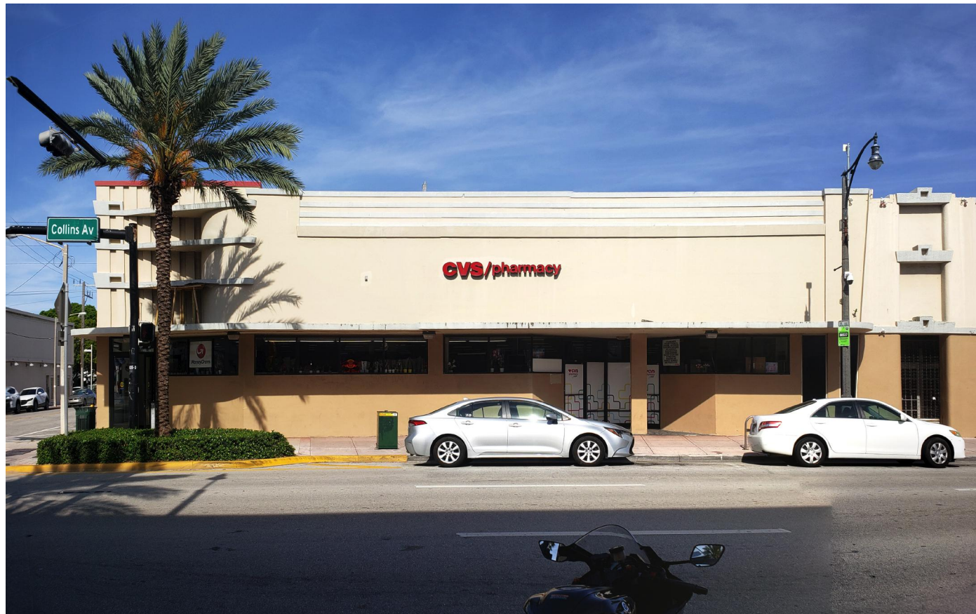
14. COLLINS AVE - EXISTING CVS
