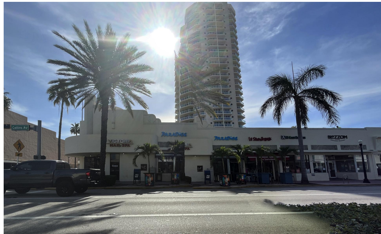
21. COLLINS AVE - STREET MALL
