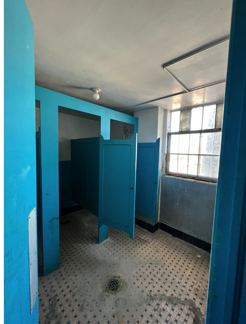
7. Restrooms at Mezzanine Level
