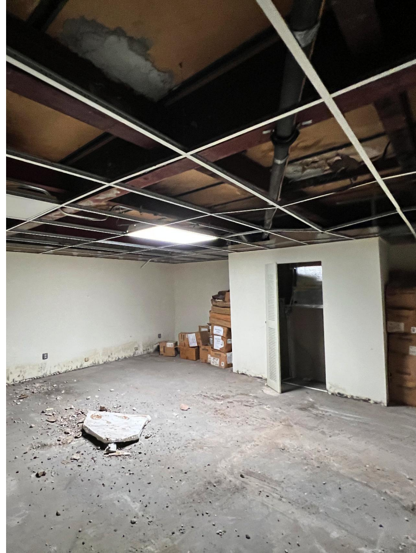
8. Interior at Mezzanine Level
