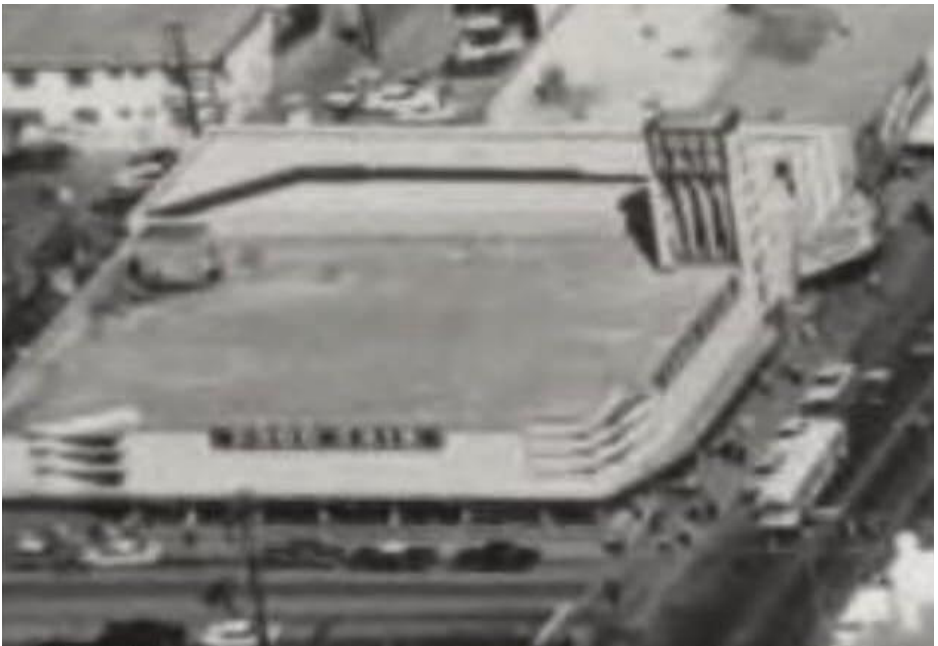
Aerial View of Food Fair Building 1950s
