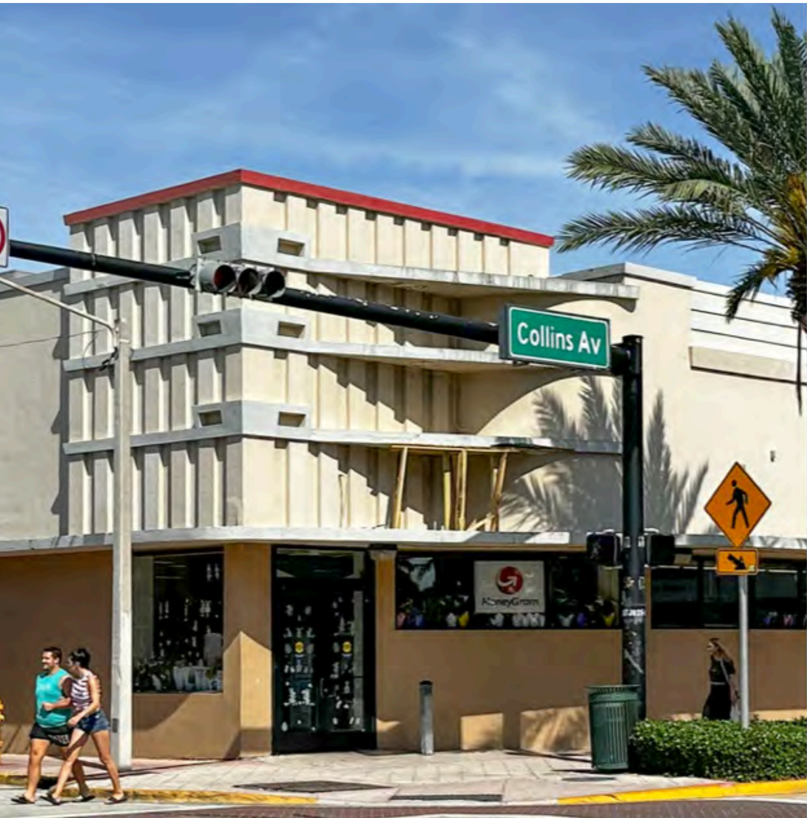
DETAIL VIEW OF CORNER ENTRANCE. NOTE THAT MOST OF THE SOUTH ELEVATION ORIGINALLY HAD THE TALLER GLASS WINDOWS ALONG THE ENTIRE SOUTH ELEVATION. THESE DEEPER WINDOWS WERE ALSO ORIGINALLY INSTALLED ALONG COLLINS AVENUE SIMILAR TO THE ONE REMAINING WINDOW ADJACENT TO THE CORNER ENTRANCE.
