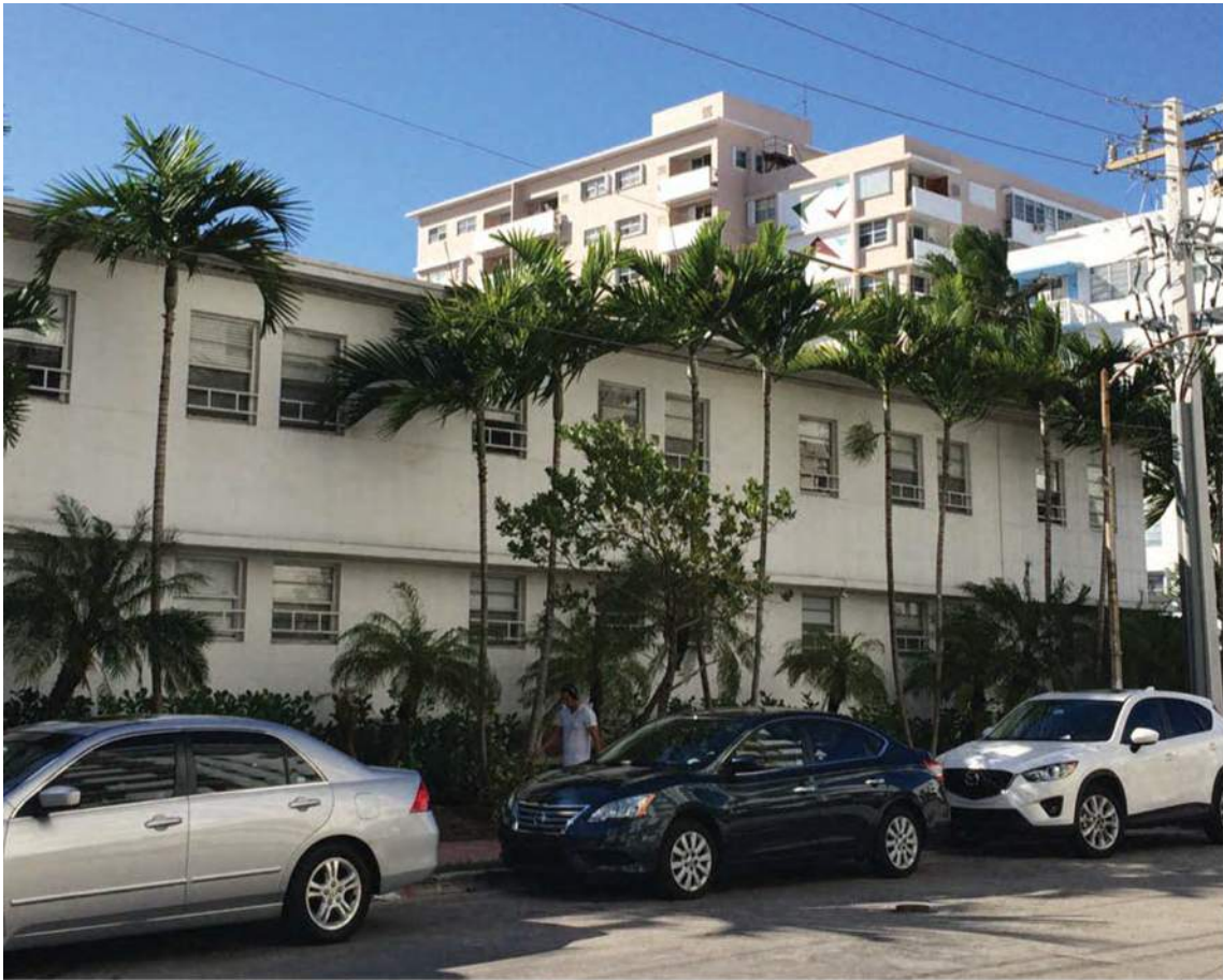
NORTH FACADE (18TH STREET)
