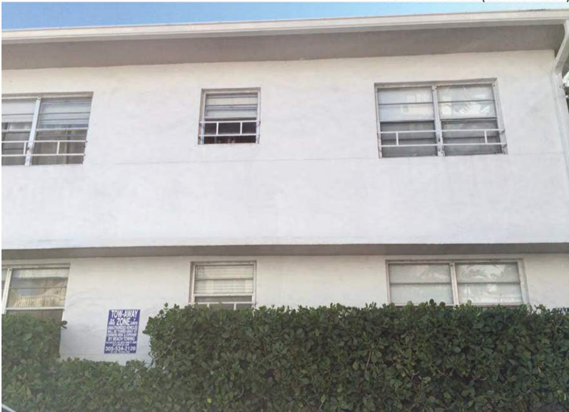
WINDOWS FACING JAMES AVENUE
