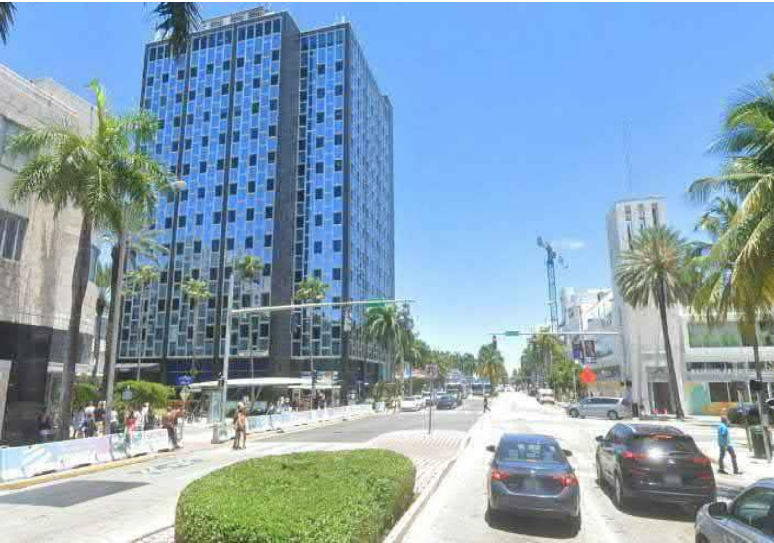
WASHINGTON AVE NORTH VIEW
