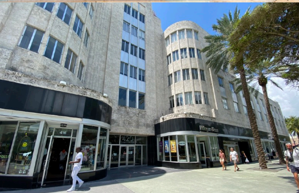
TOP PHOTO: RITZ CARLTON DiLIDO HOTEL MIDDLE PHOTO: 818 LINCOLN ROAD LOWER PHOTO: 420 LINCOLN ROAD
