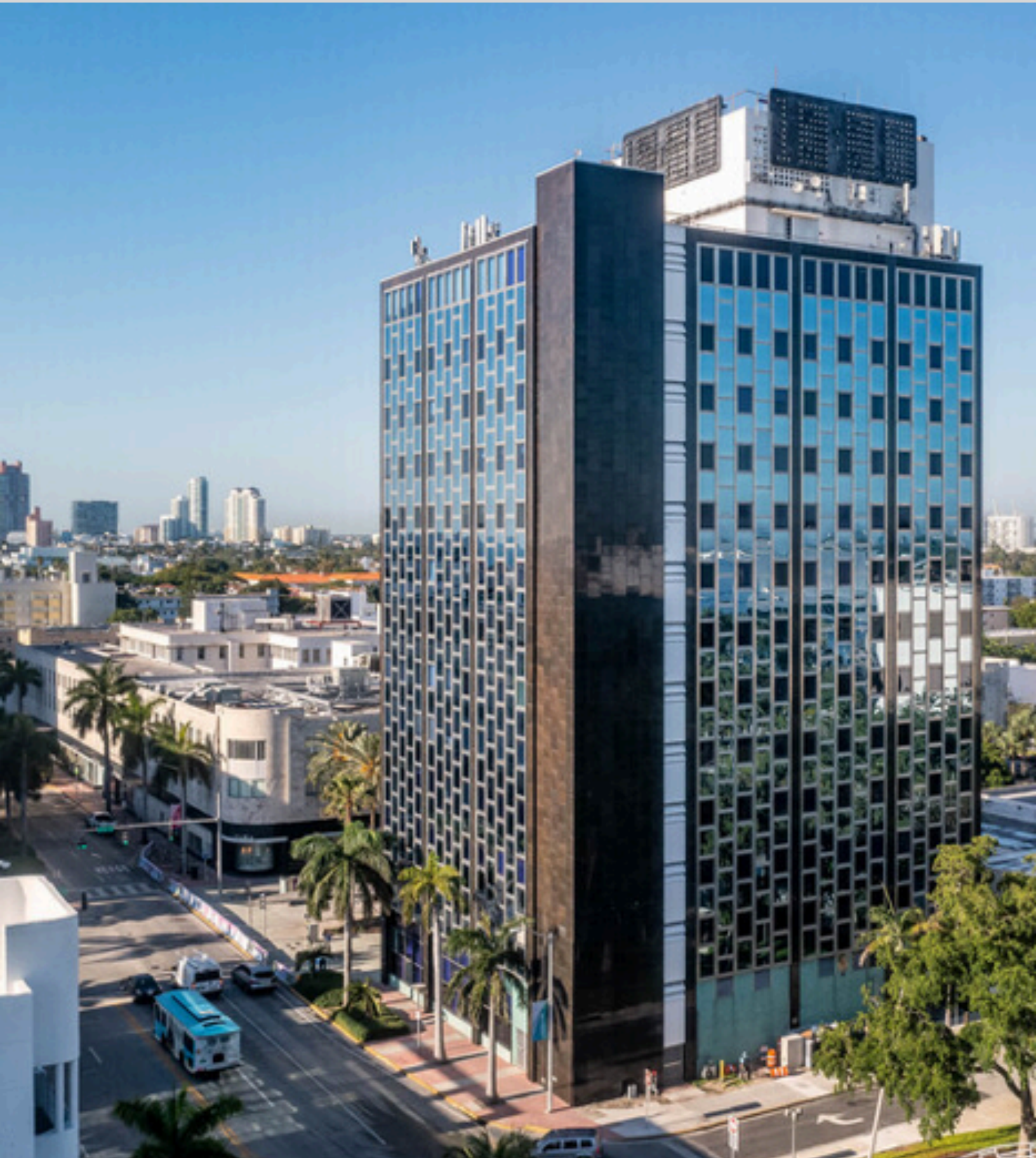
AERIAL VIEW LOOKING SOUTHWEST TOWARDS 407 BUILDING FROM WASHINGTON AVENUE (4)
