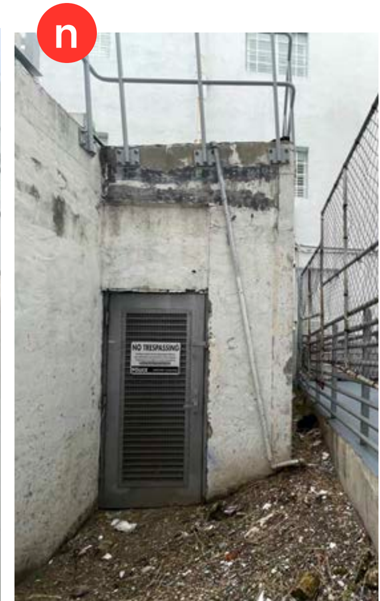
DOOR TO EXISTING BOILER ROOM
