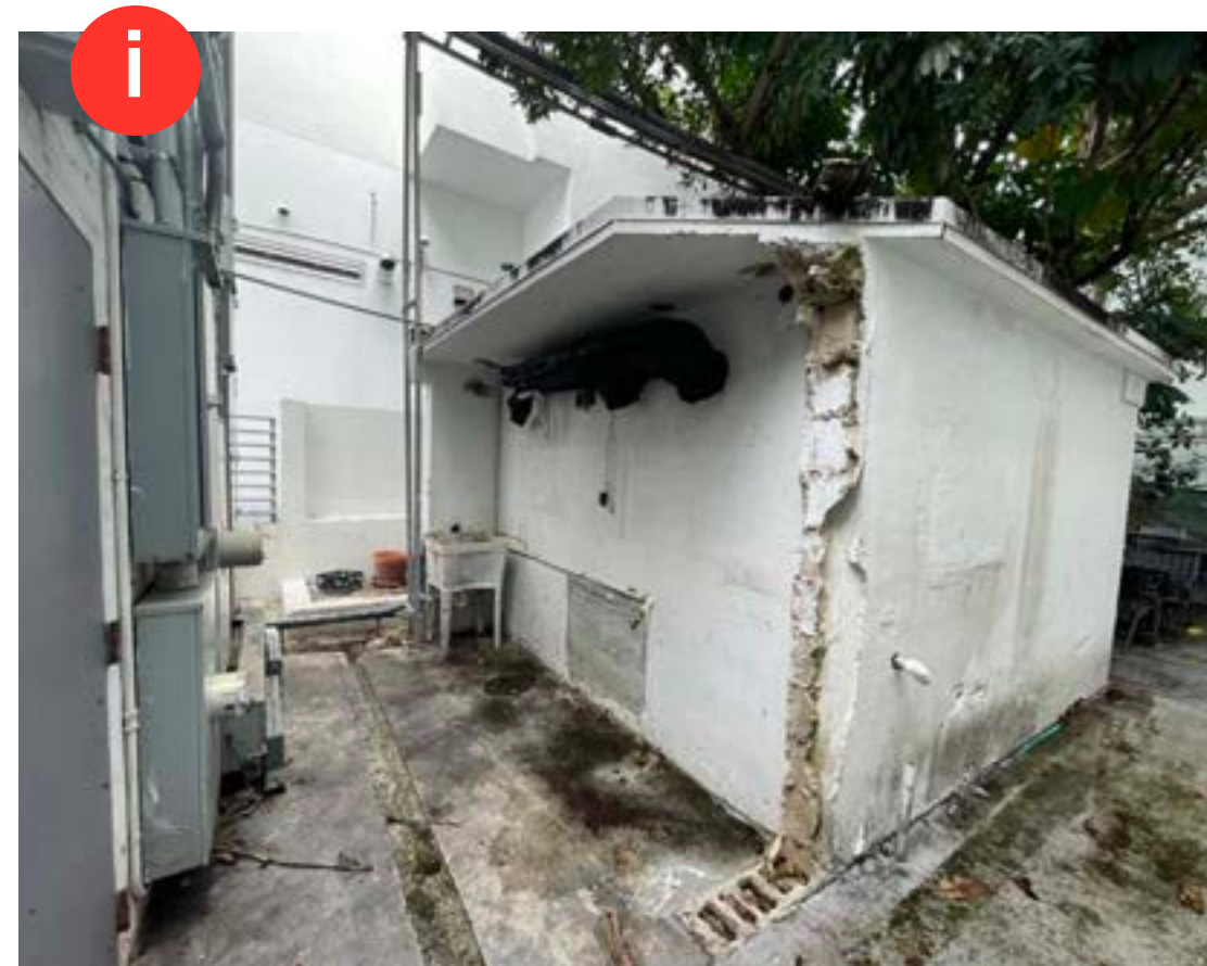
CORNER VIEW OF EXISTING STORAGE ROOM - NORTHEAST VIEW
