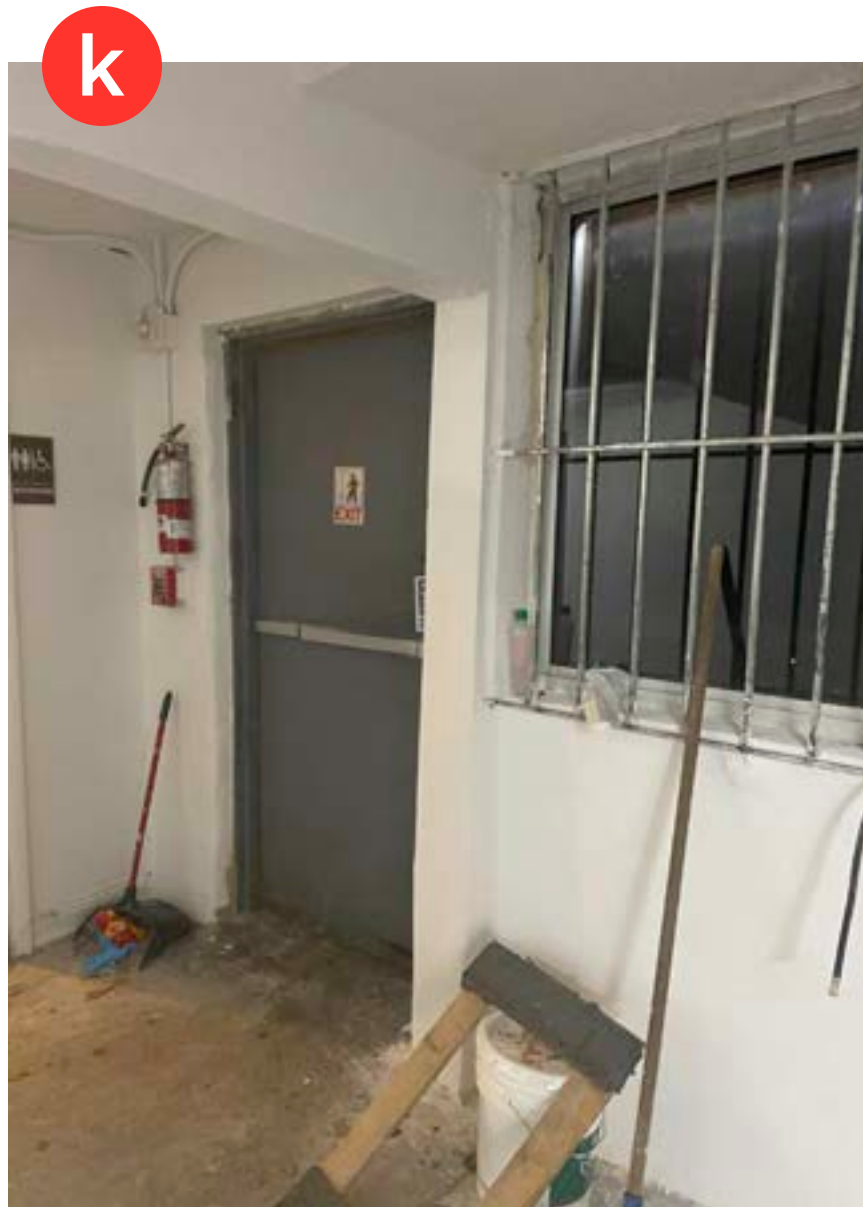
VIEW OF UNOCCUPIED TENANT SPACE (NON-CONTRIBUTING ADDITION PORTION)
