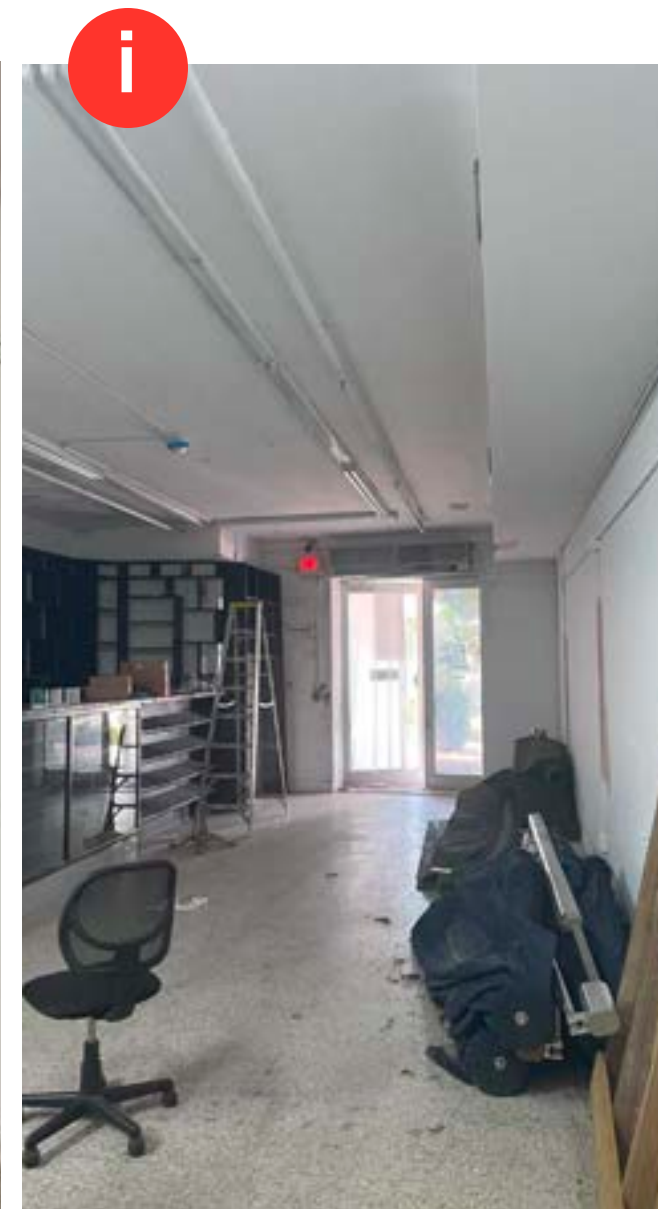
VIEW BACK TOWARD ENTRANCE OF THE UNOCCUPIED TENANT SPACE (FACING WEST)
