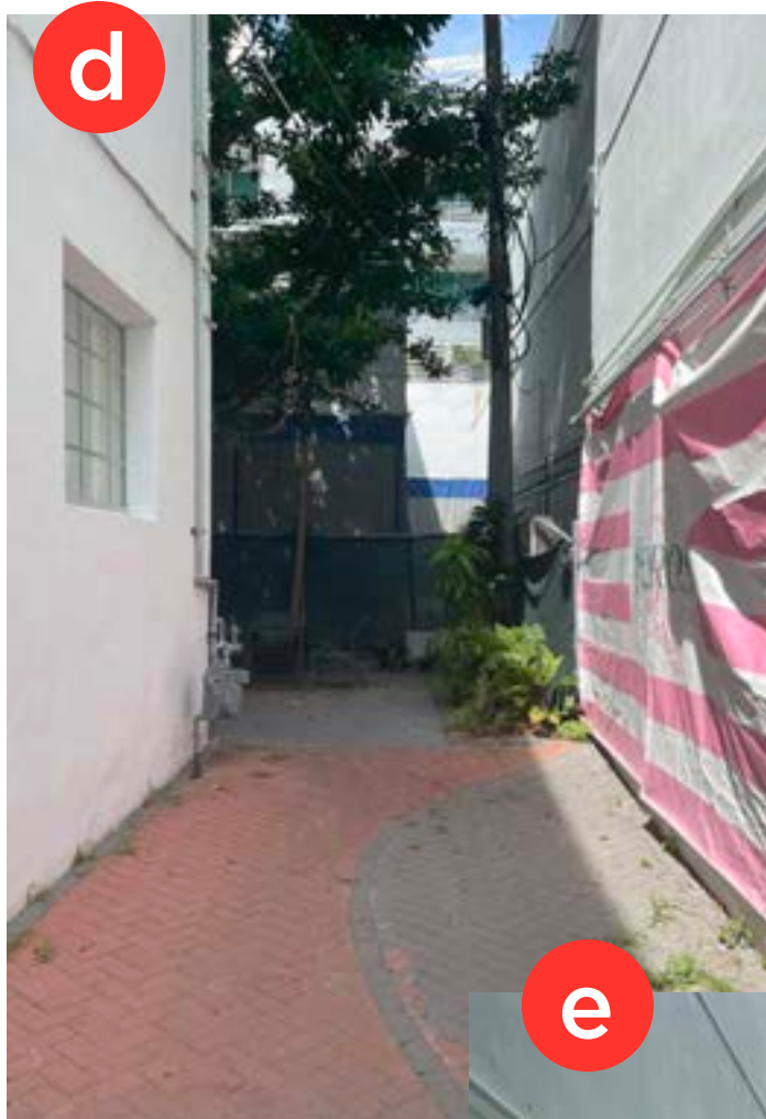
REAR PROPERTY VIEW ADJACENT TO ALLEY FACING NORTH
