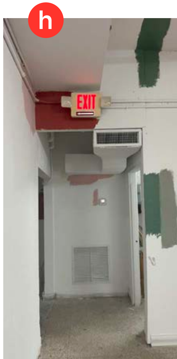
VIEW UPON ENTERING UNOCCUPIED TENANT SPACE (FORMER HOTEL CARD ROOM & KITCHEN)
