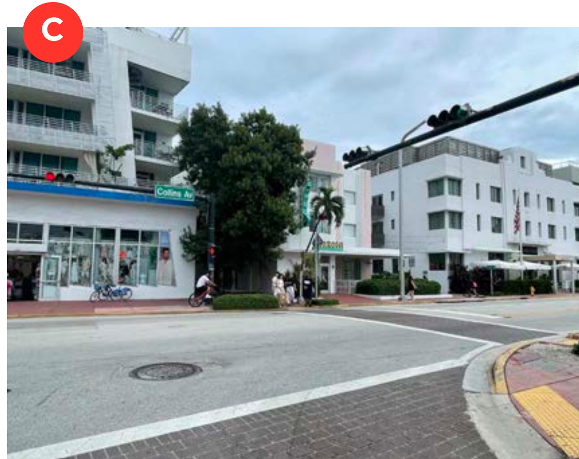
COLLINS AVE AT ESPANOLA WAY - SOUTHEAST VIEW (Z OCEAN HOTEL ON LEFT, HENROSA HOTEL IN MIDDLE, BETSY HOTEL ON RIGHT)
