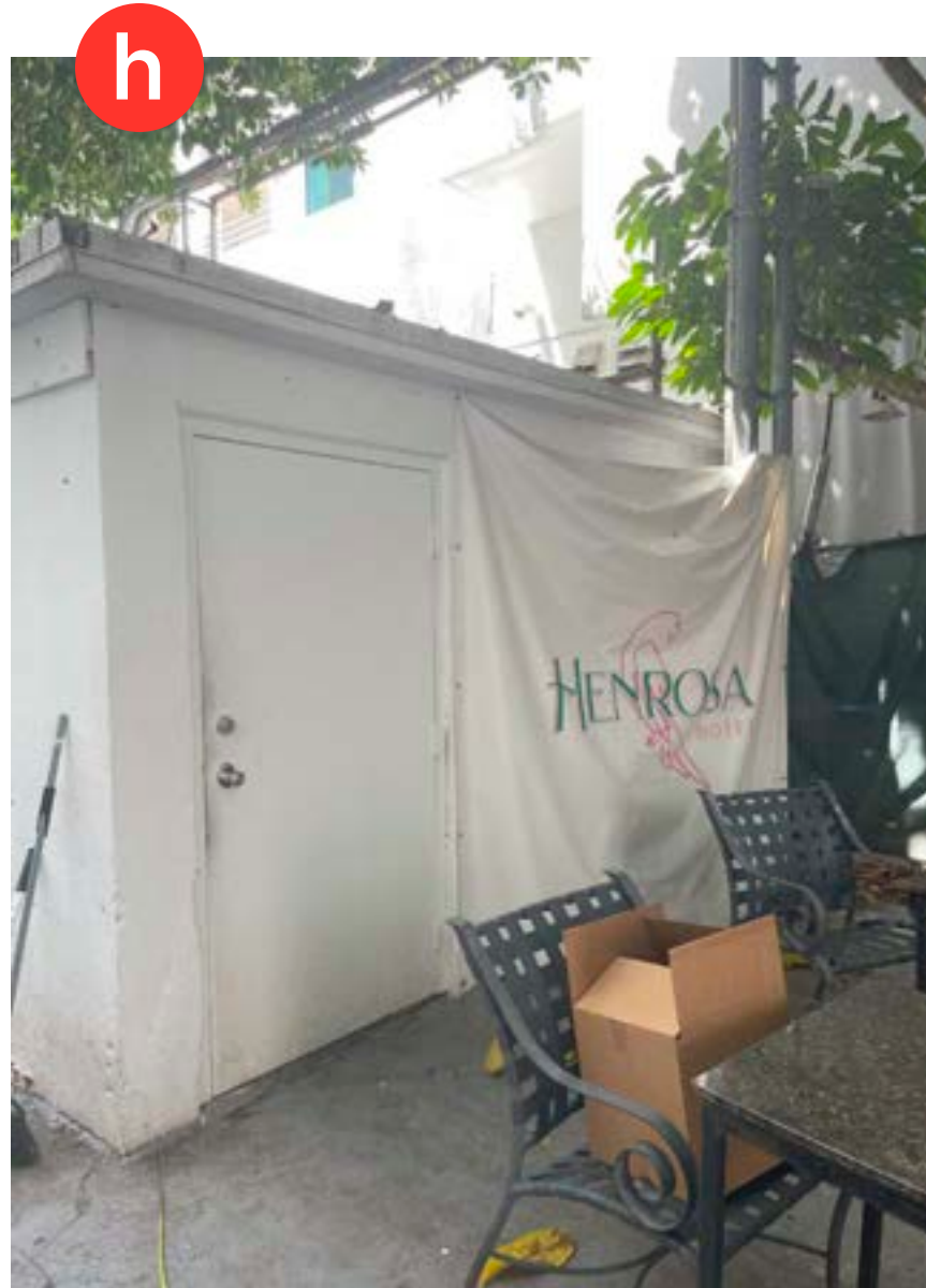
EXISTING STORAGE ROOM EAST WALL (PROPOSED OUTDOOR BAR STRUCTURE LOCATION)
