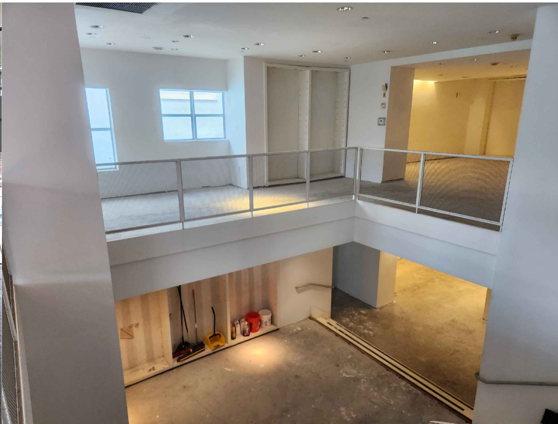
C4 INTERIOR OF THE BUILDING: VIEW TO THE MAIN HALL FROM THE 2ND FLOOR LEVEL PHOTO TAKEN: 06-20-2023
