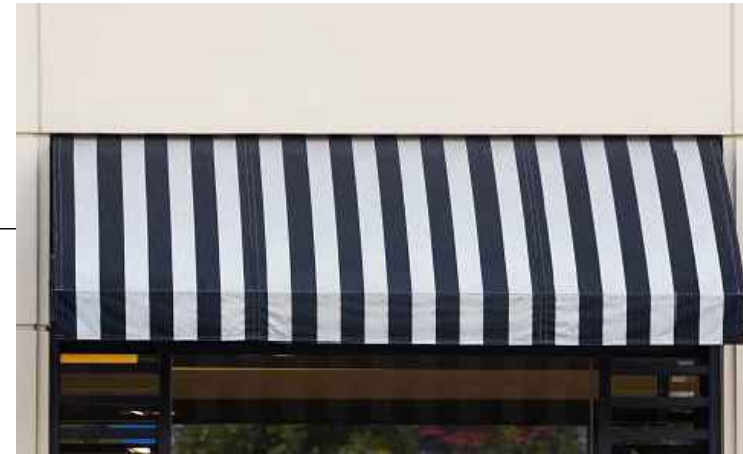
A2 BLACK AND WHITE STRIPED CANVAS AWNING OVER THE STOREFRONT AT MAIN FACADE.
