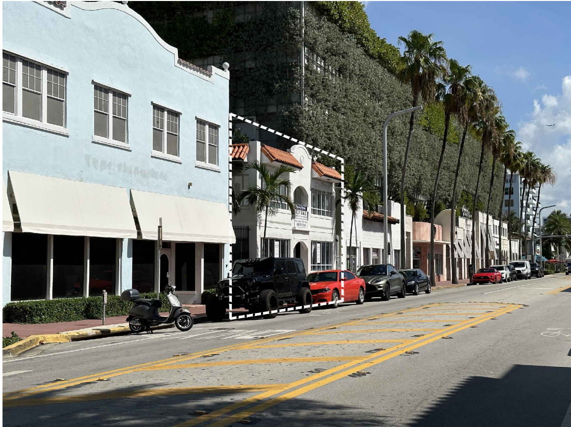
A1 VIEW FROM WESTERN SIDEWALK ON COLLINS AVE. INTERCEPTION WITH 6TH STREET PHOTO TAKEN: 06-20-2023
