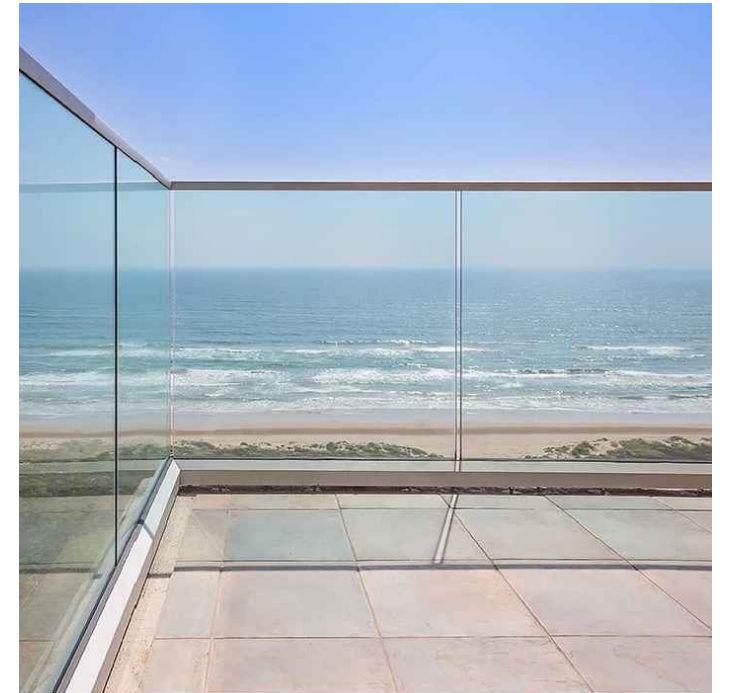
A3 NEW 42" HEIGHT FRAMELESS GLASS GUARDRAIL AT ROOFTOP AND STAIRCASE.
