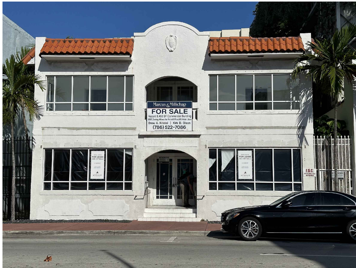
C1 BUILDING MAIN FACADE (FRONTAGE AT COLLINS AVENUE) PHOTO TAKEN: 06-20-2023
