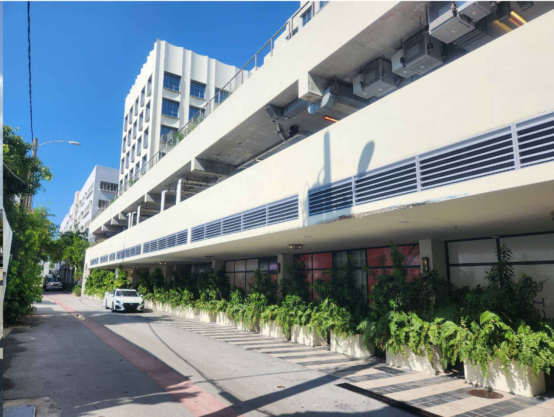
A4 VIEW FROM THE REAR OF THE BUILDING AT THE ALLEY TOWARDS 6TH STREET PHOTO TAKEN: 06-20-2023
