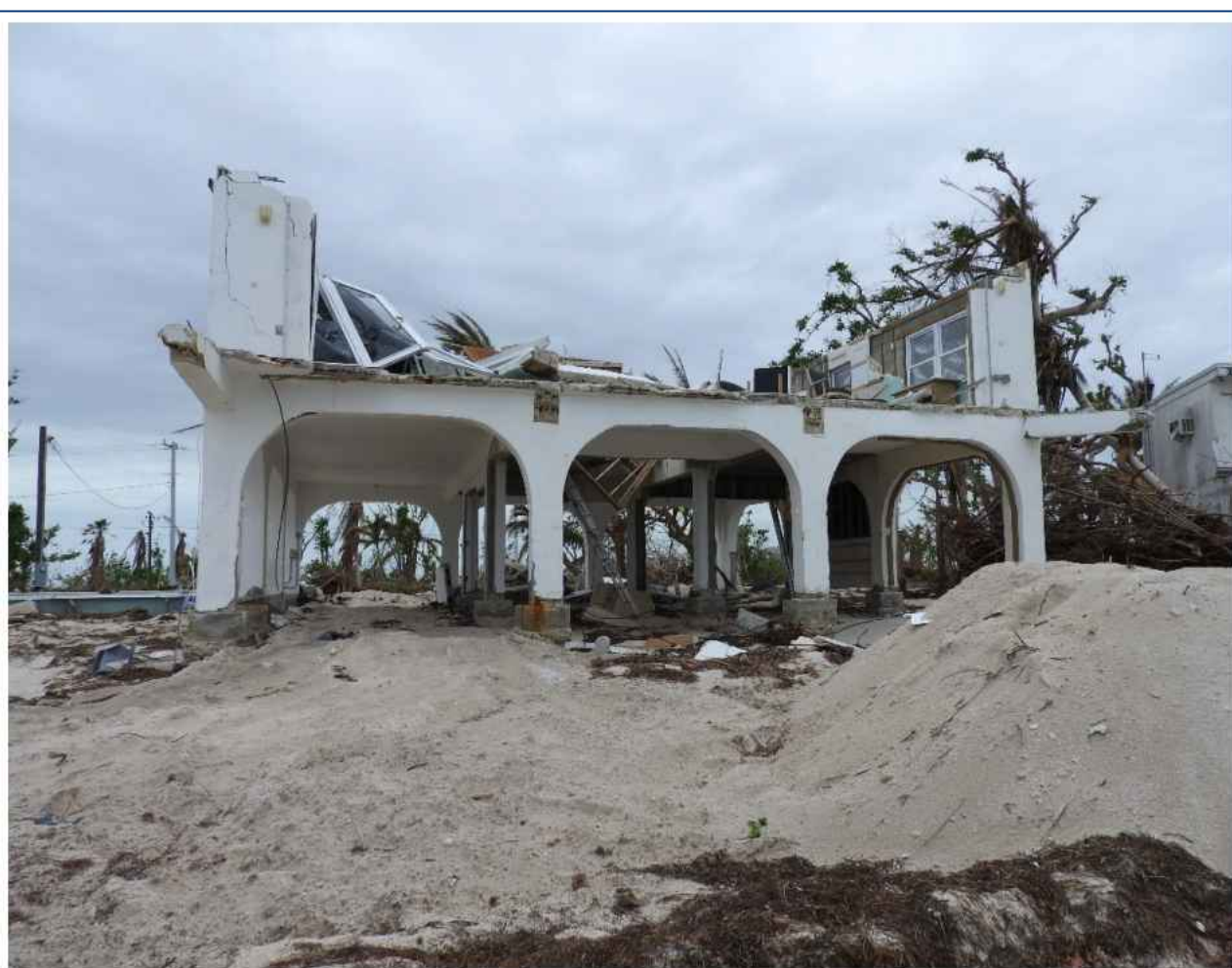
Figure 91. Single-family dwelling destroyed, Long Beach, Big Pine Key.
