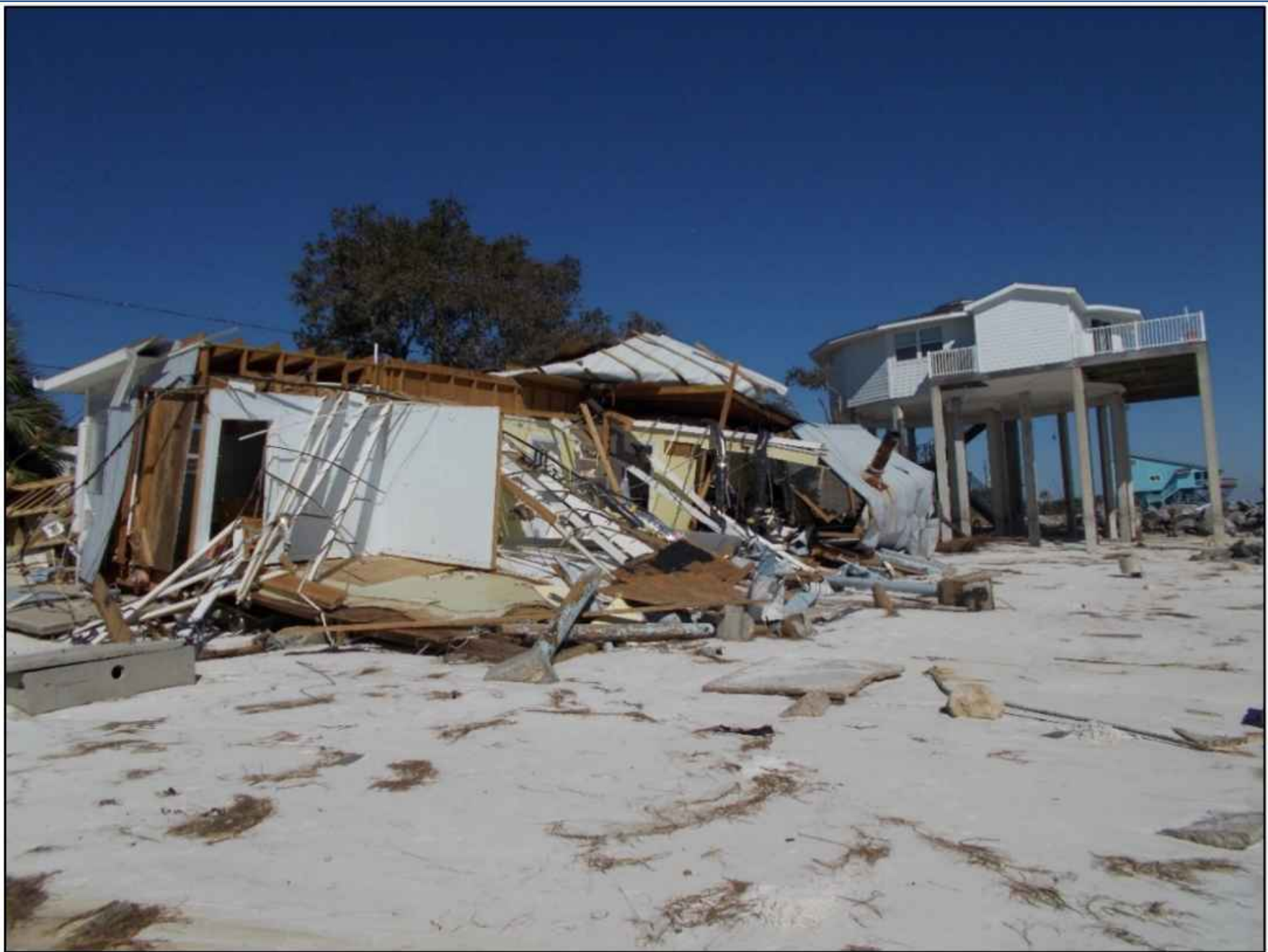
Figure 101. Dwelling destroyed near R211, Southwest Cape.
