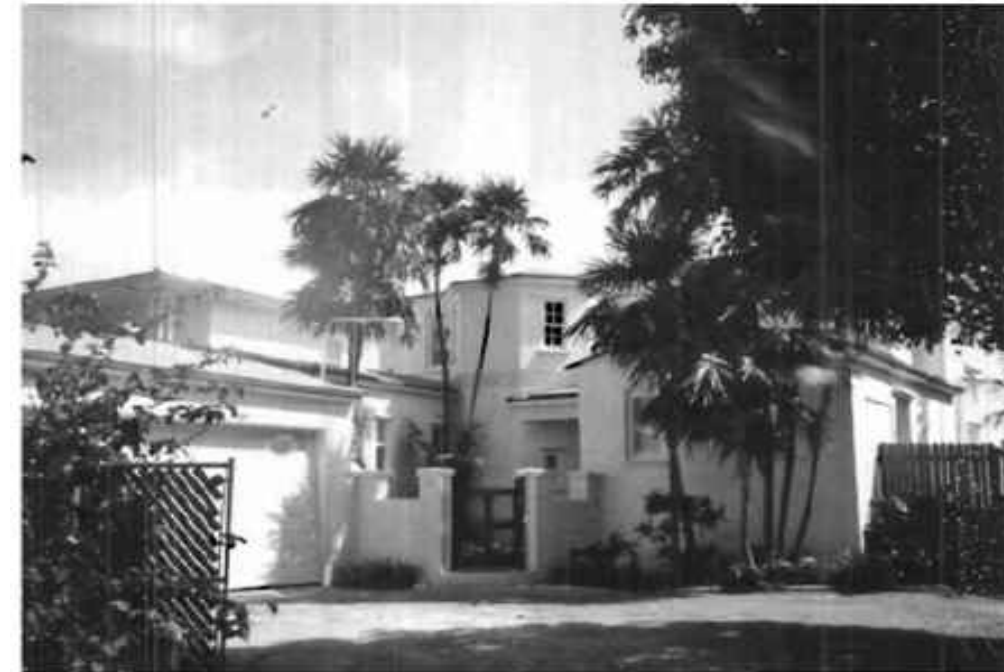
Figure 43. View of front façade of 7801 Atlantic Way, February 1995. (Office of the Property Appraiser, Miami-Dade County)
