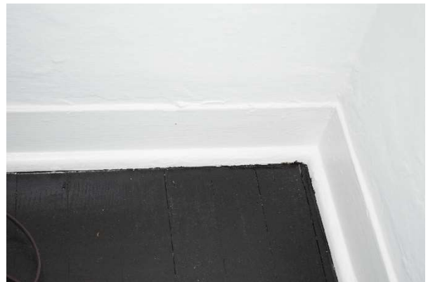
Figure 21. Wood base and flooring at Bedroom 1, May 2021.
