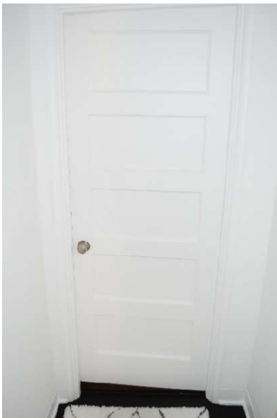
Figure 30. Interior door at Hall, May 2021.
