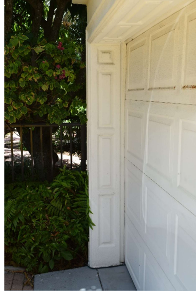
Figure 12. Garage door casing, May 2021.
