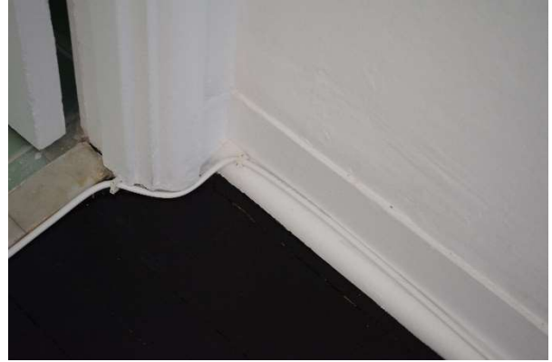
Figure 33. Wood base at Bedroom 3, May 2021.
