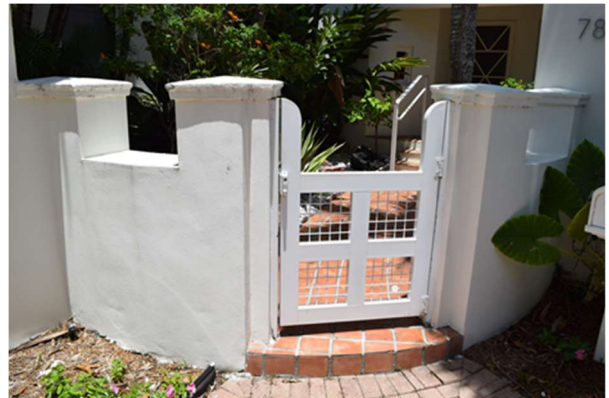
Figure 2 Wood gate adjacent driveway, May 2021.
