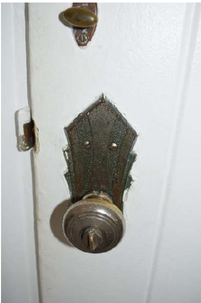
Figure 5. Front door interior hardware, May 2021.
