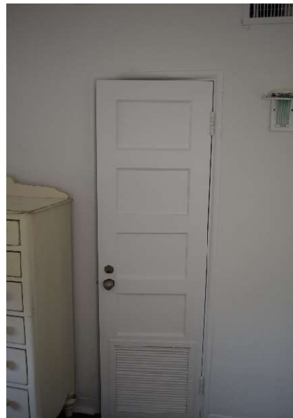
Figure 38. Interior closet door at Bedroom 4, May 2021.
