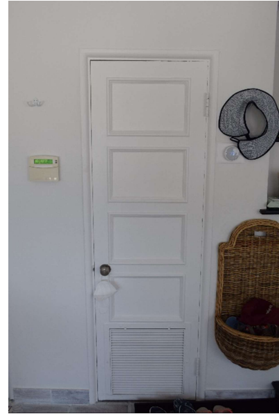
Figure 16. Interior door at Living Room, May 2021.
