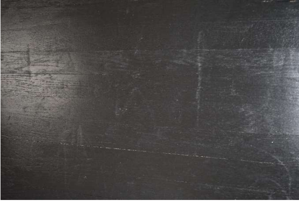
Figure 39. Wood flooring at Bedroom 4, May 2021.
