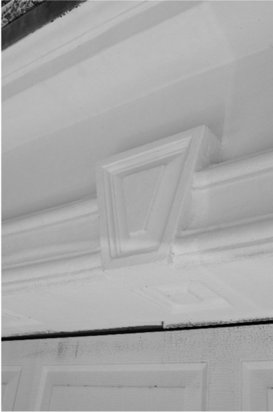
Figure 11. Garage door trim, with keystone, May 2021.
