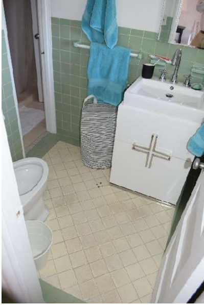
Figure 35. Floor and wall tile at Bath 3, May 2021.
