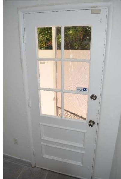
Figure 14. Exterior side door, May 2021.
