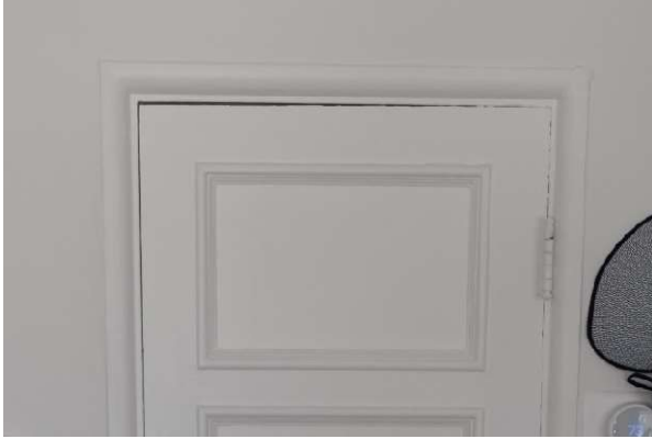
Figure 19. Trim at interior doors, May 2021.
