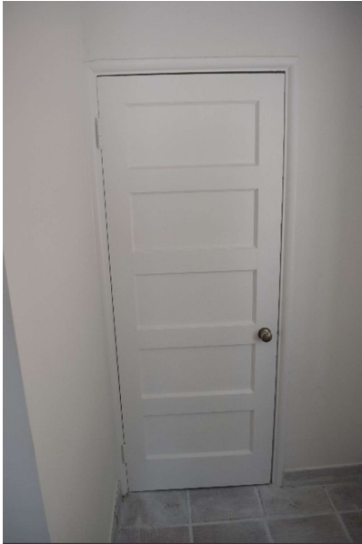
Figure 15. Interior door at Living Room, May 2021.
