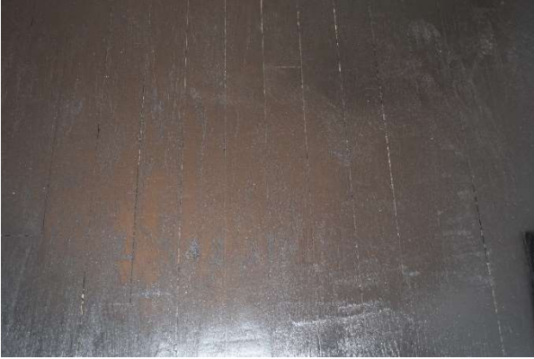
Figure 32. Wood flooring at Bedroom 3, May 2021.
