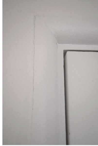
Figure 23. Interior door trim at Bedroom 1, May 2021.
