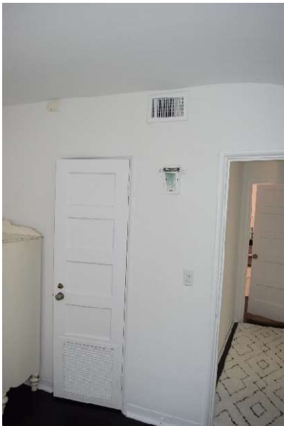
Figure 37. Interior door at Bedroom 4, May 2021.
