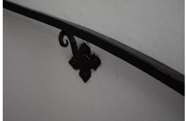
Figure 29. Bracket supporting stair handrail, May 2021.
