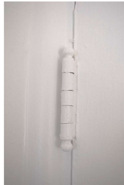
Figure 18. Hinge at interior door, May 2021.
