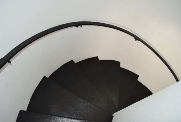
Figure 28. Stair handrail, May 2021.
