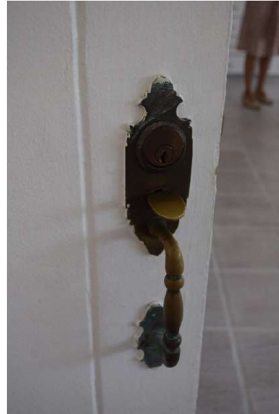
Figure 4. Front door exterior hardware, May 2021.
