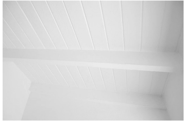
Figure 8. Tongue & groove ceiling at front porch, May 2021.
