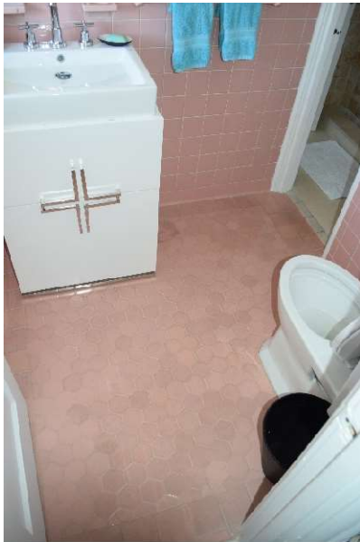
Figure 41. Floor and wall tile at Bath 4, May 2021.
