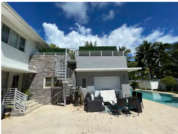
Photo 5 – Garage & Rooftop Deck
