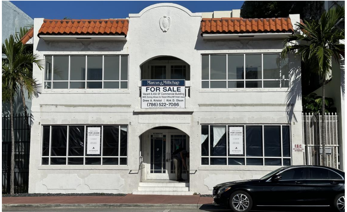
EXHIBIT (I): FRONT BUILDING FAÇADE (EAST ELEV.) / PHOTO TAKEN: June 20, 2023
