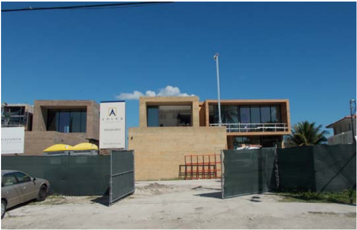
W 825 E DI LIDO DRIVE UNDER CONSTRUCTION
