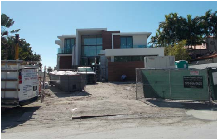
Y 8 W RIVO ALTO DRIVE UNDER CONSTRUCTION
