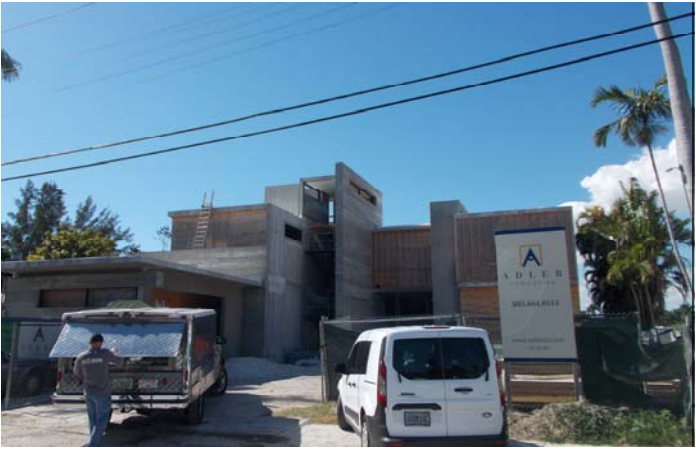
U 122 W DI LIDO DRIVE UNDER CONSTRUCTION
