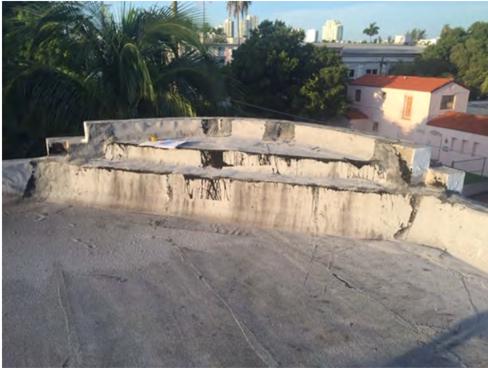
South West Roof pylon support
