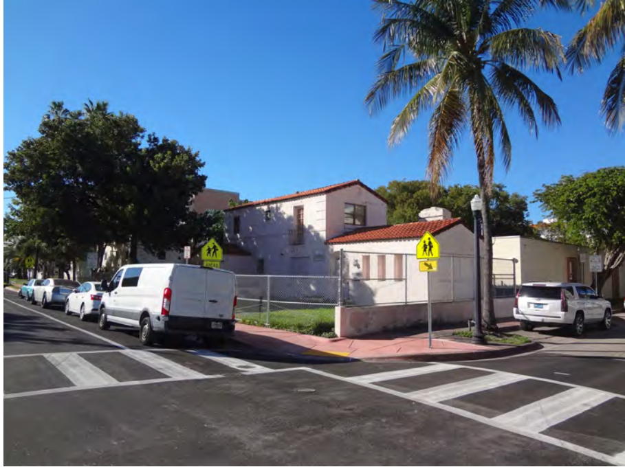
South West across street
