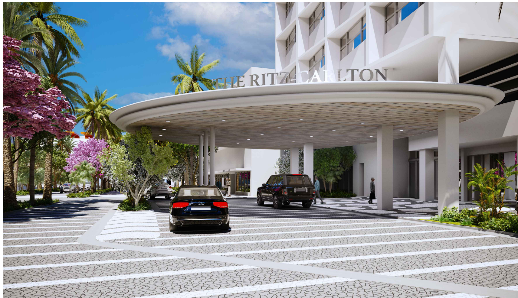
RITZ CARTLON VALET DROP OFF CANOPY
