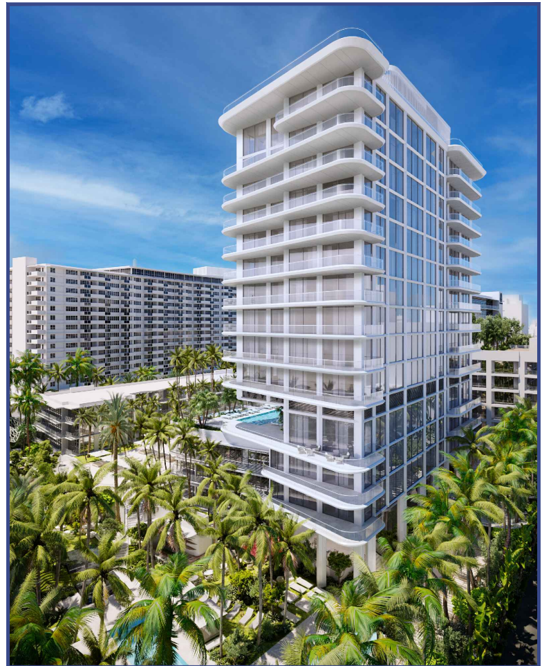
8. Ground Up Addition
