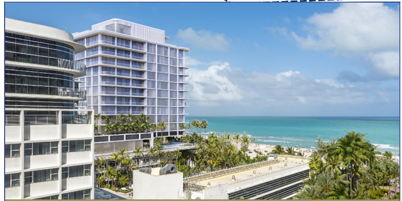
7. Ground Up Addition
