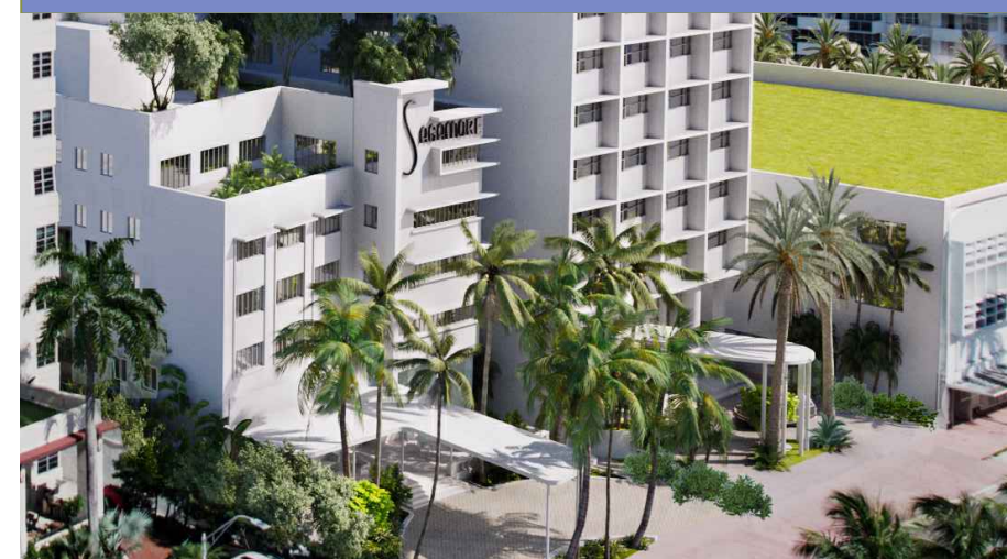
Sagamore Facade - Terrace Restoration
