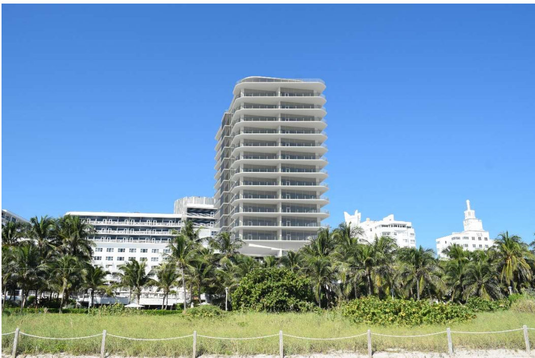
Figure 28. Rendered view depicting 2021 proposed tower behind Sagamore Hotel. (Heritage Architectural Associates with K4 Architecture)
