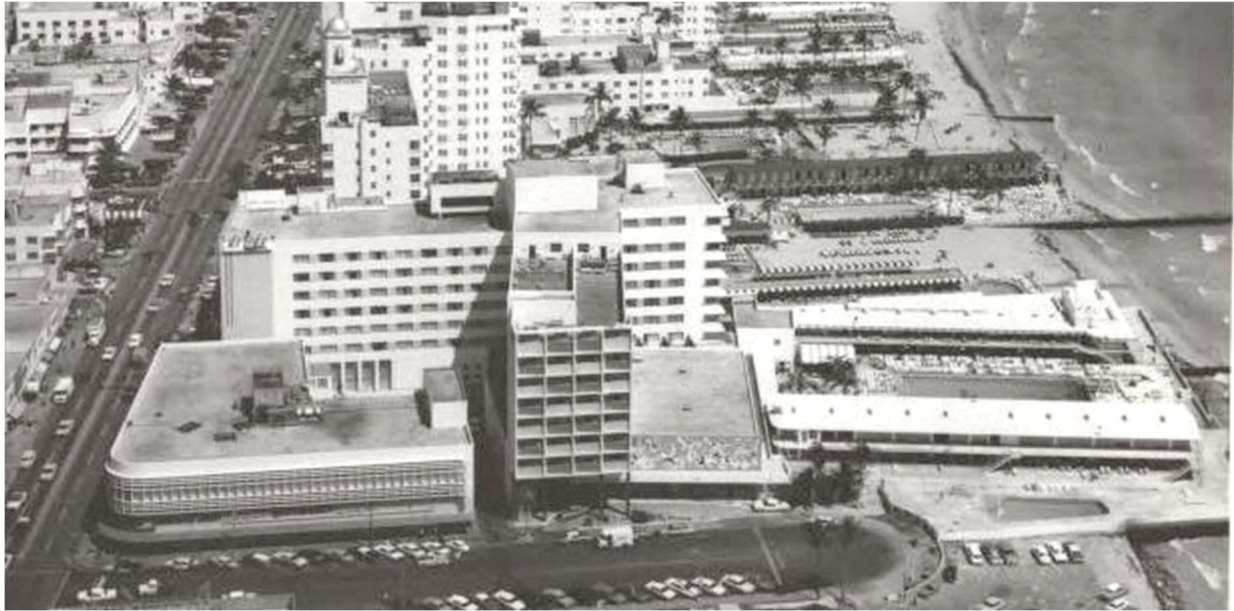
Figure 1. Former DiLido Hotel and Wolfie's Building, c. 1962. (FIU Libraries)
