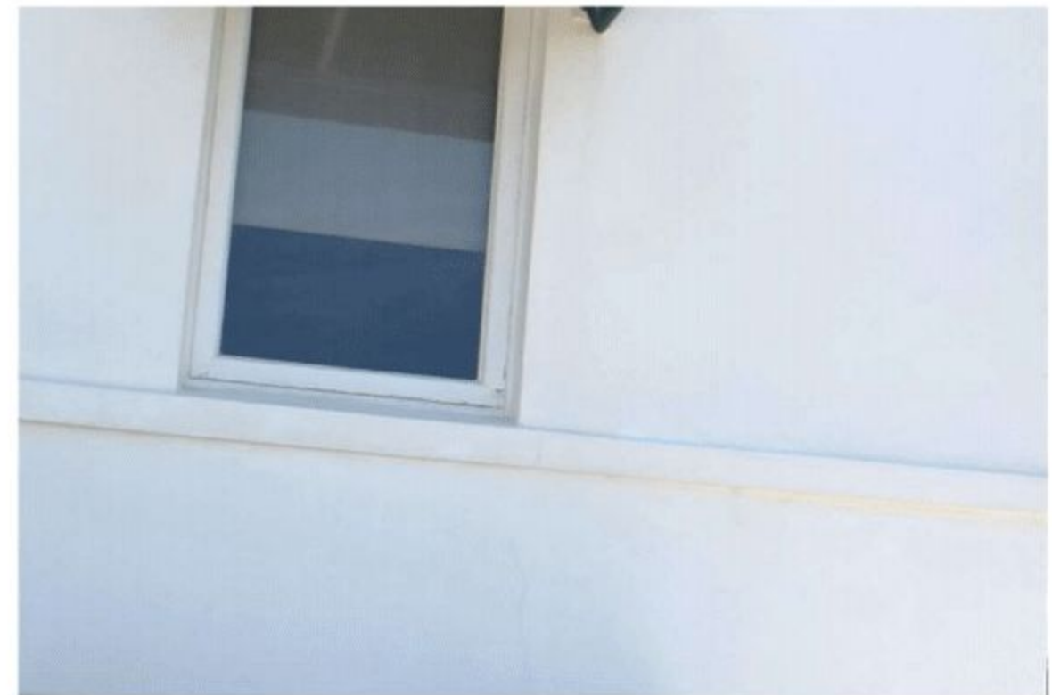
Figure 85. Detail of belt course below second story windows, May 2021.
