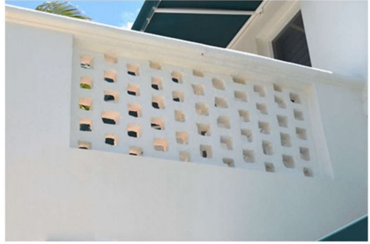
Figure 83. Detail of breezeblock at veranda, May 2021.
