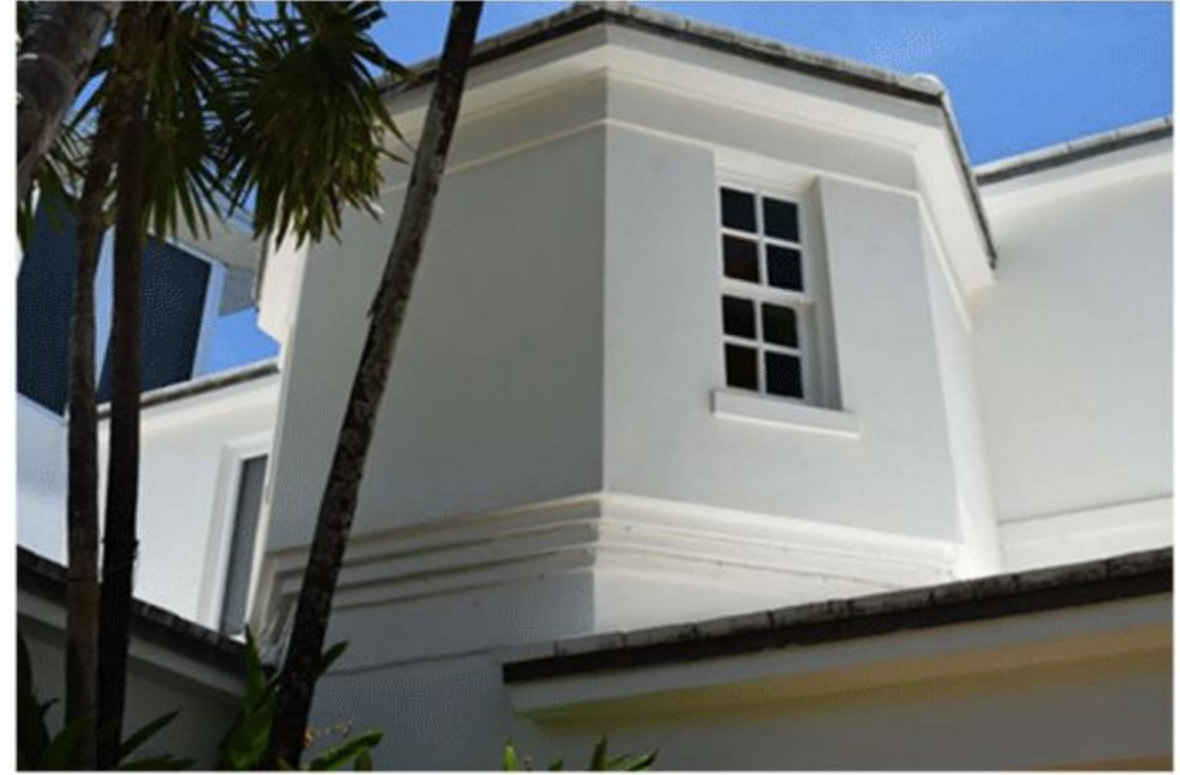
Figure 75. Detail of octagonal stair tower with cornice and corbelled detailing, May 2021.
