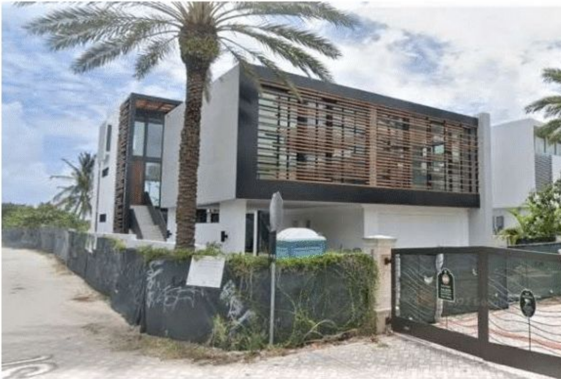
Figure 28. 7845 Atlantic Way (under construction), July 2022. (©Google Street View)
