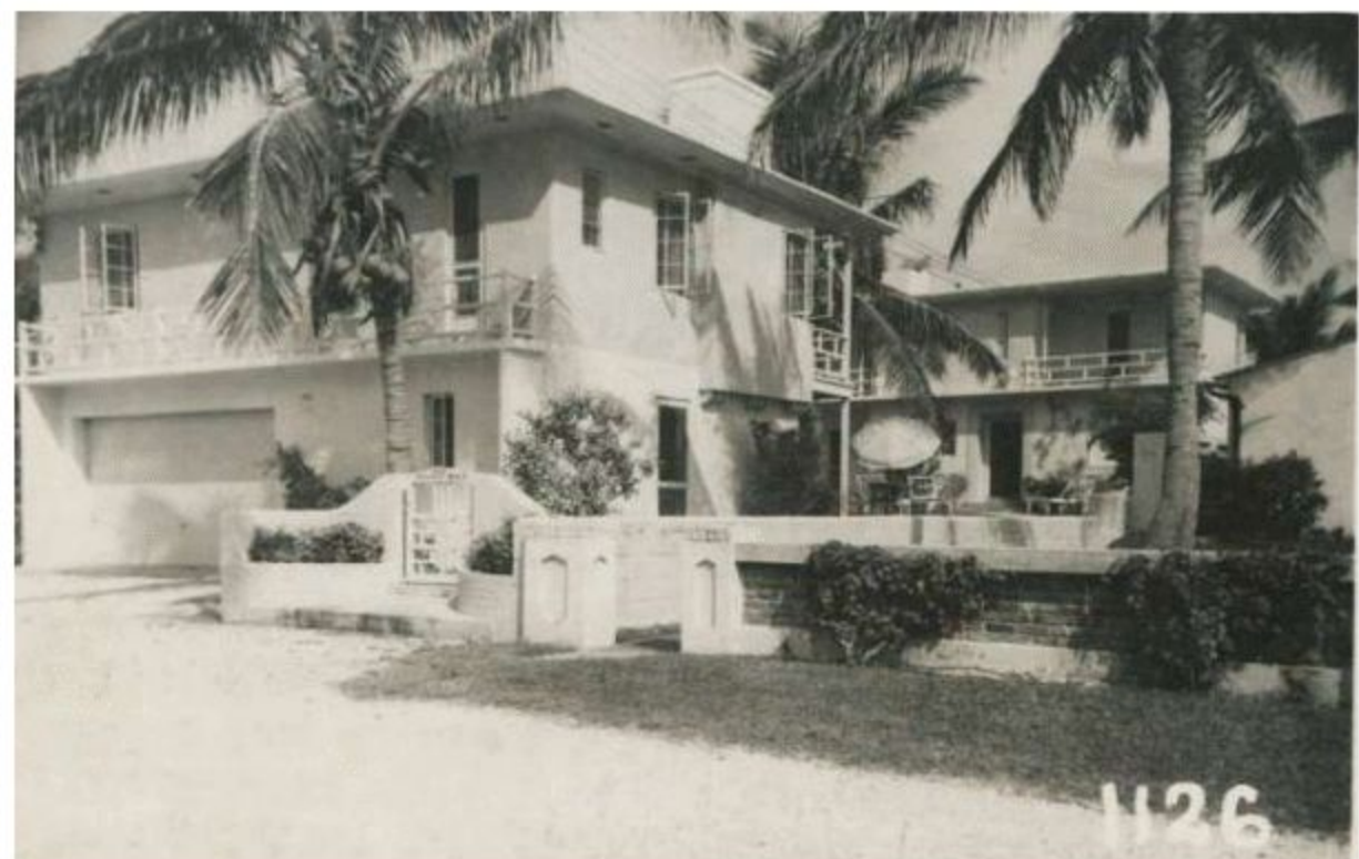
Figure 33. 7815 Atlantic Way (constructed 1936), October 1947. (Miami-Dade Public Library)
