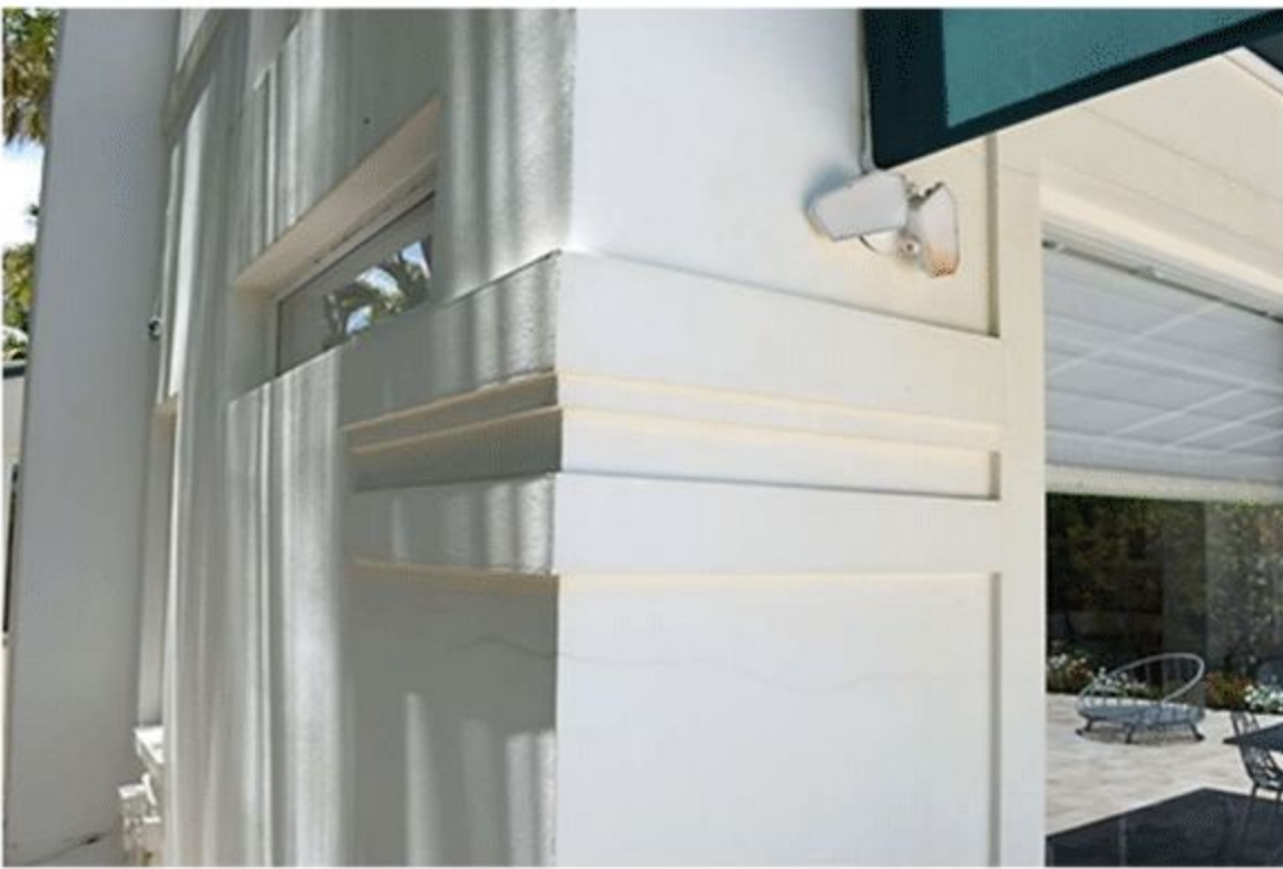
Figure 84. Detail of paired horizontal molding, May 2021.
