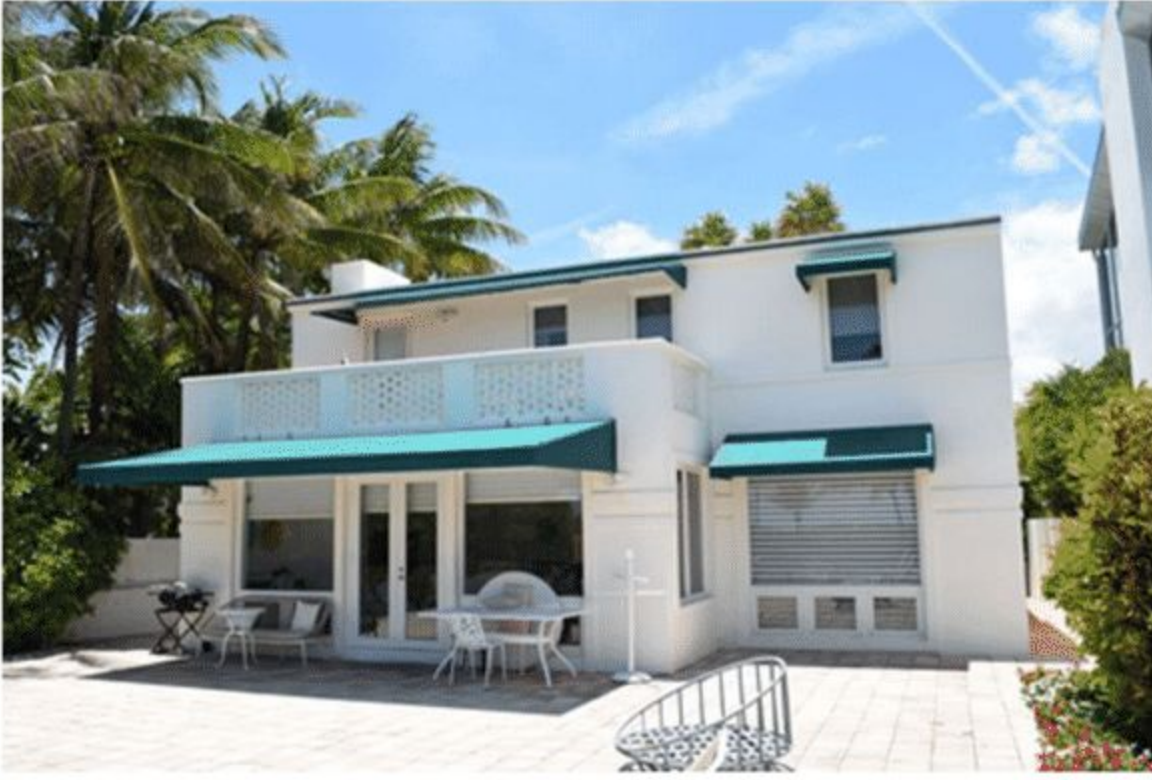
Figure 82. View of east elevation with one-story enclosed porch, May 2021.
