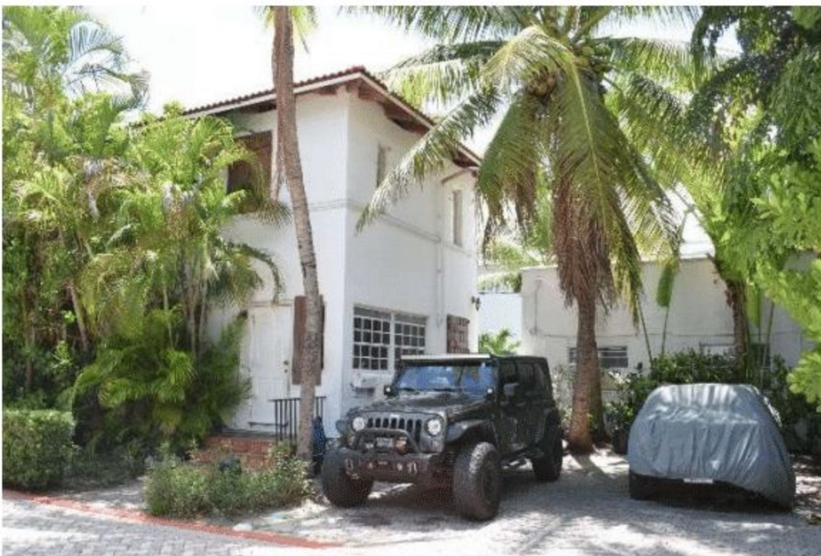
Figure 19. 101 78 th Street (constructed 1938), May 2021.
