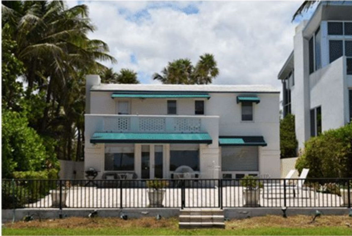
Figure 69. Patio, metal fence and steps leading to back yard, May 2021.
