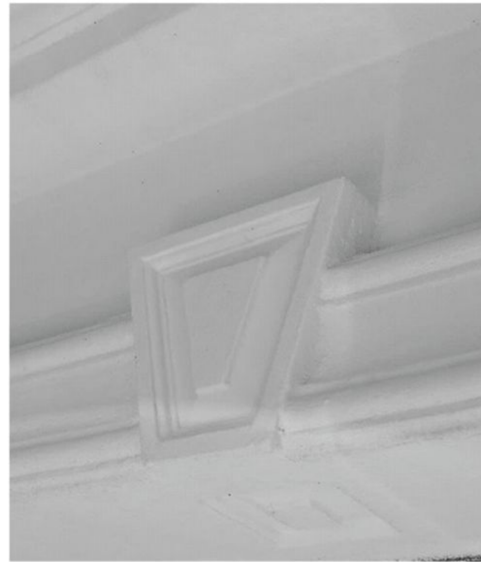
Figure 81. Detail of keystone at garage door, May 2021.
