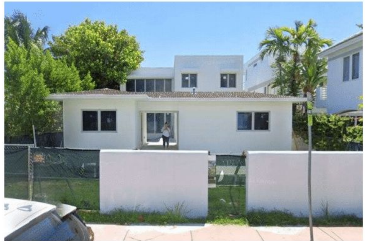
Figure 26. 7711 Collins Avenue (under construction), August 2022. (©Google Street View)
