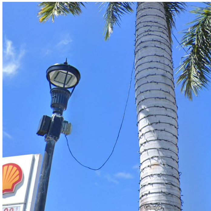
UNSAFE WIRING
