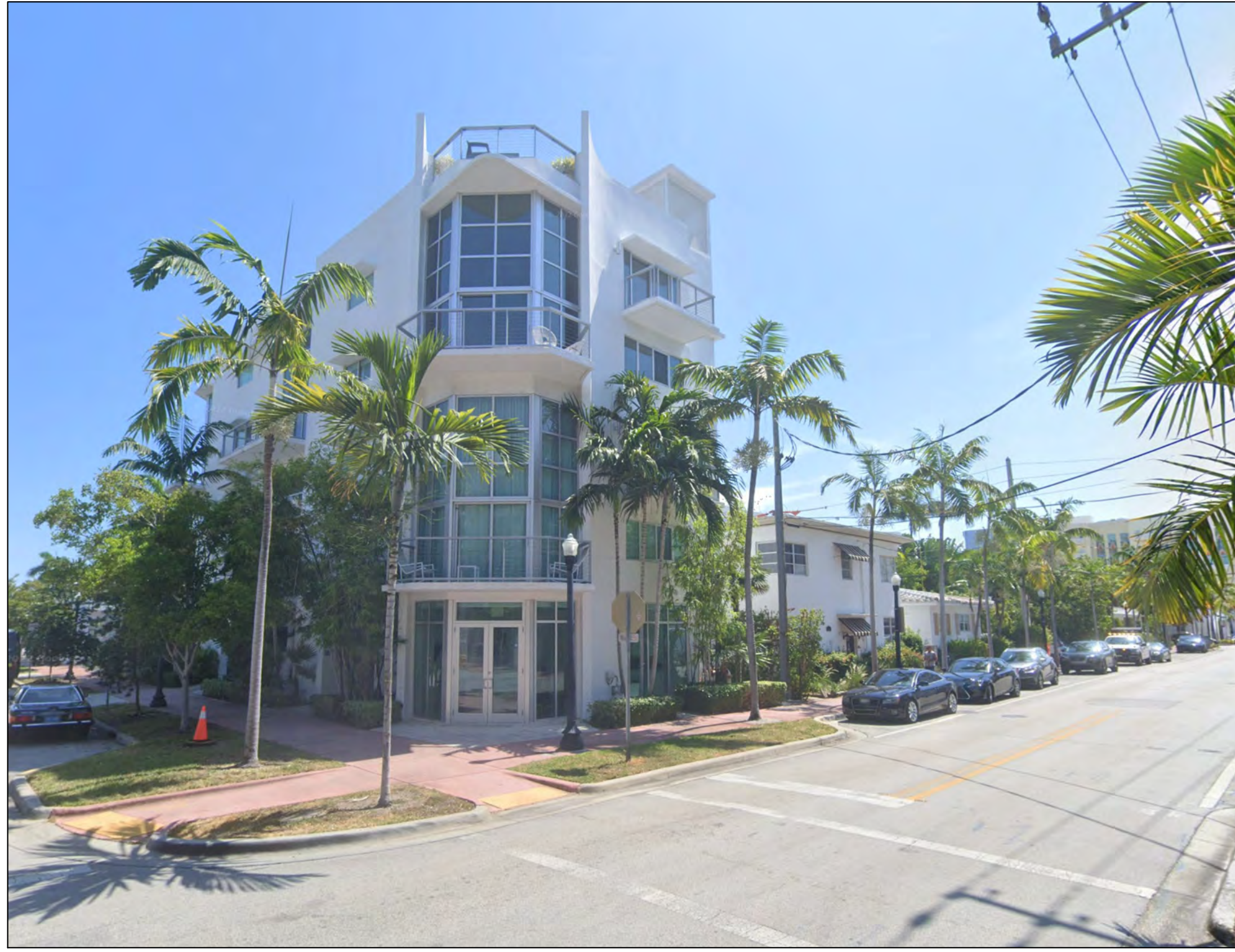
8. STREET VIEW - NORTH SIDE FACING NE
