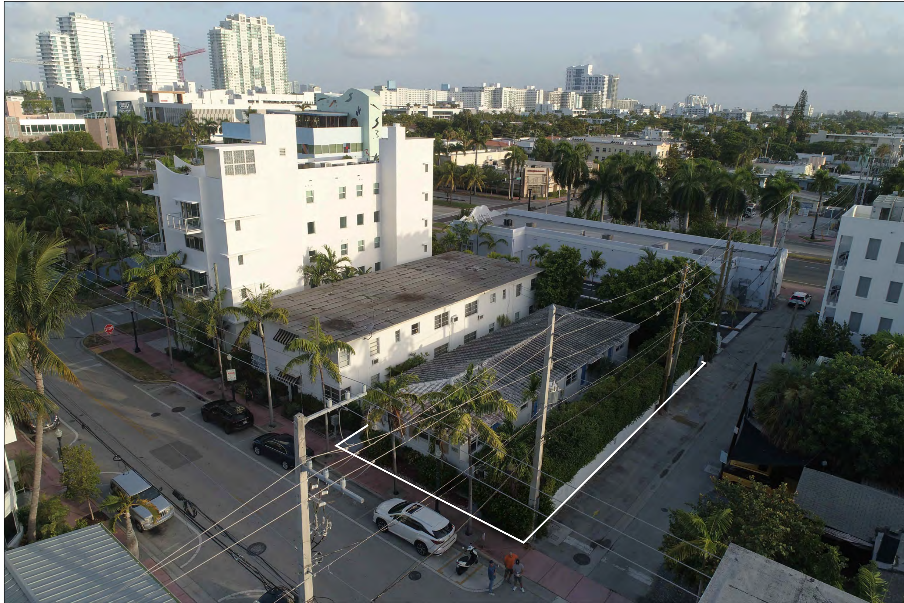
6. AERIAL VIEW OF 829 4TH STREET FACING NW
