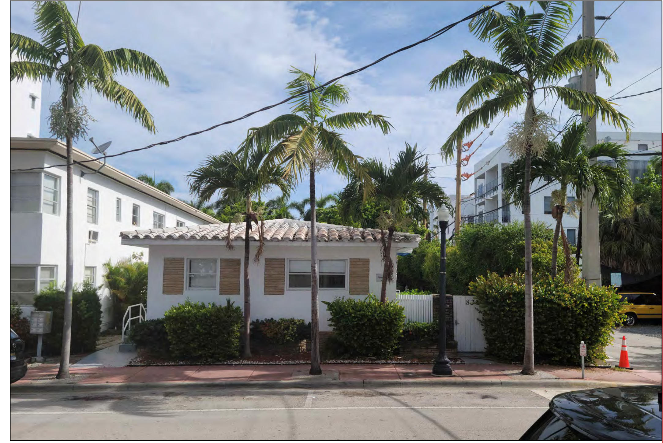
15. STREET FACADE VIEW @ 4TH STREET
