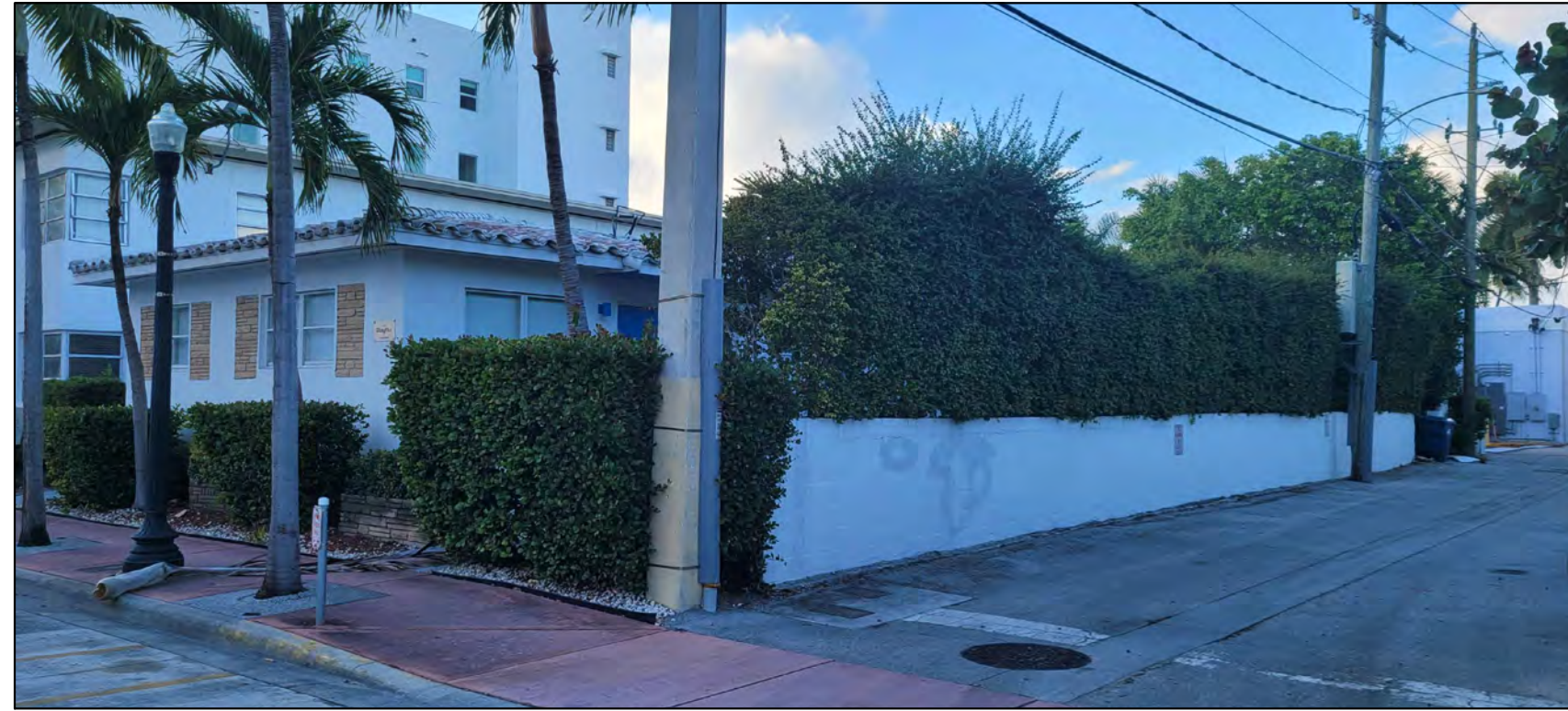
4FT CMU WALL AND HEDGE ALONG ALLEY TO BE DEMOLISHED
