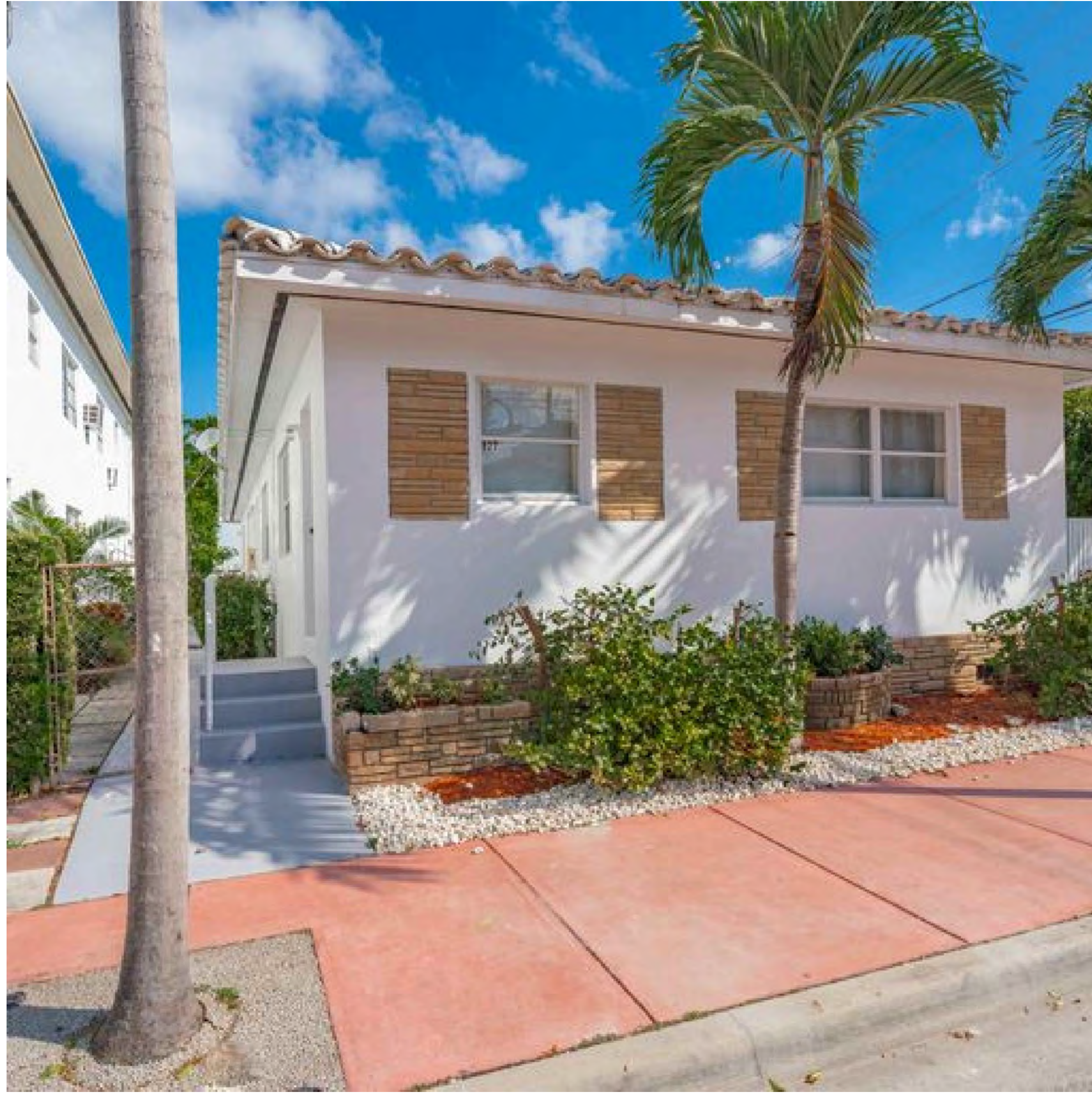
14. STREET FACADE VIEW @ 4TH STREET
