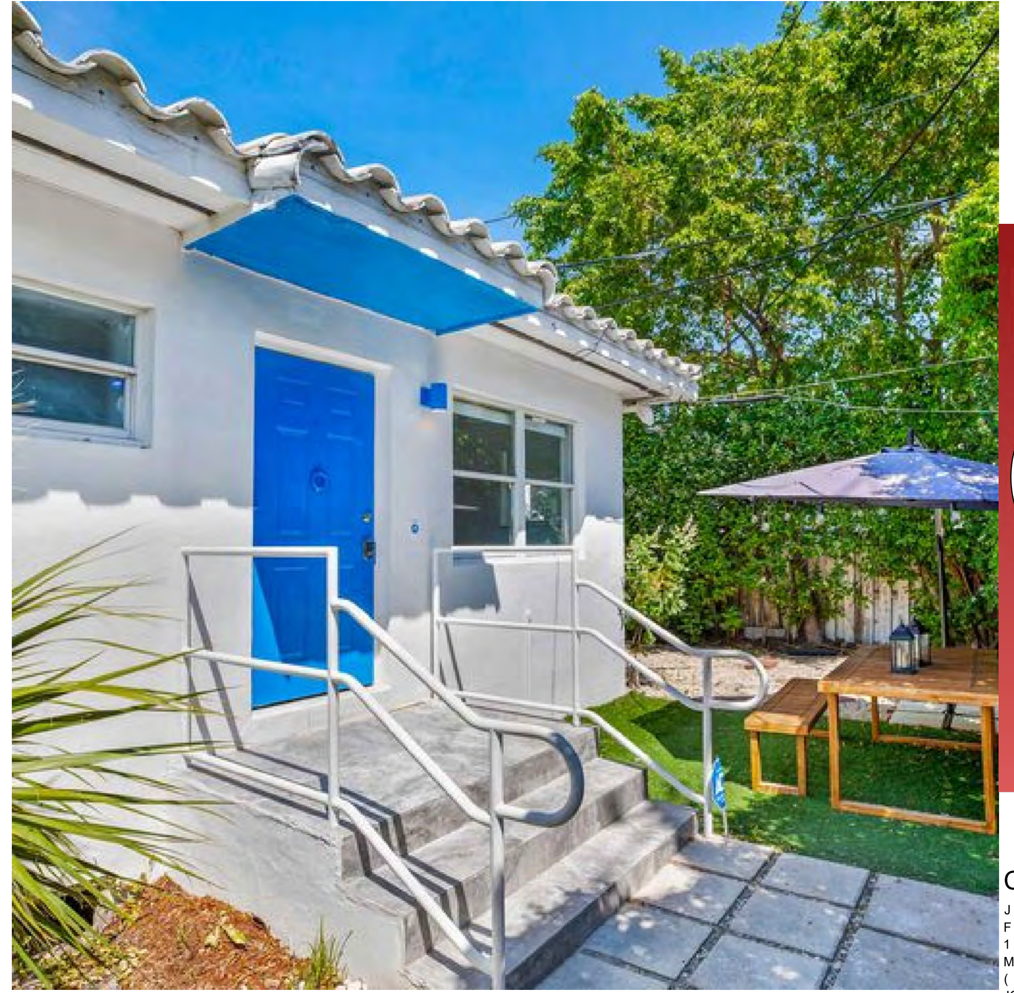
12. STAIR STOOP AND HANDRAILS
