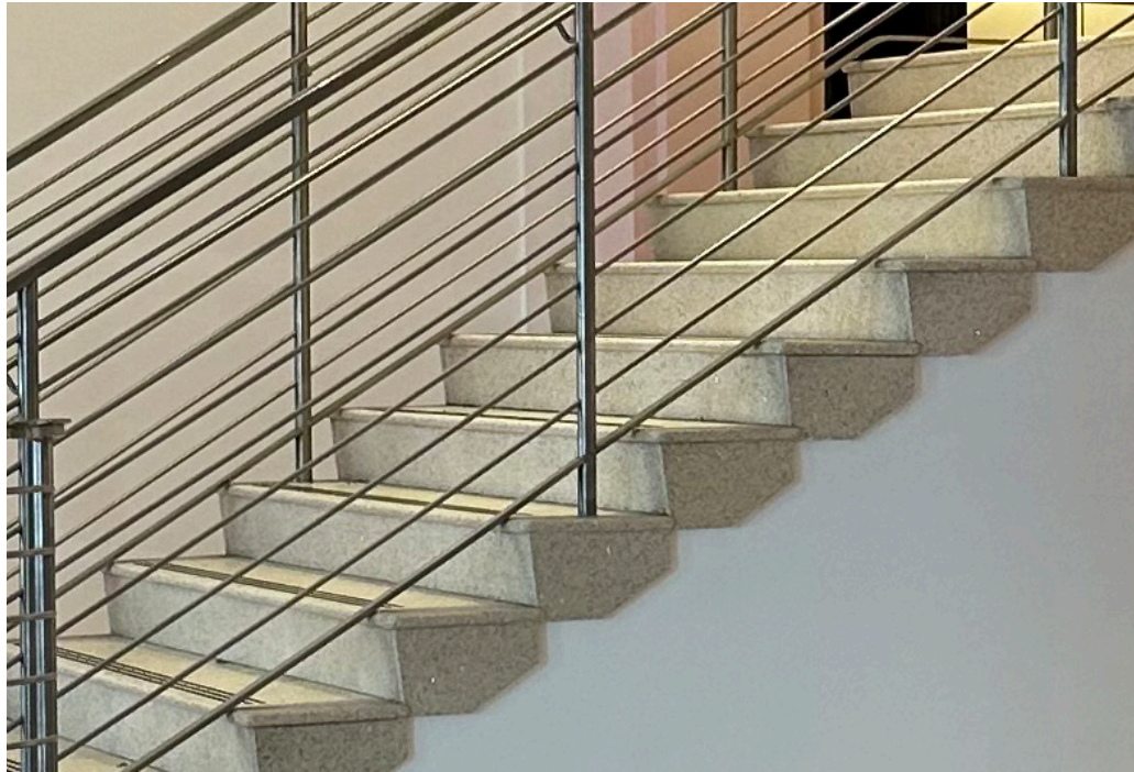
Non-historic stair detail
