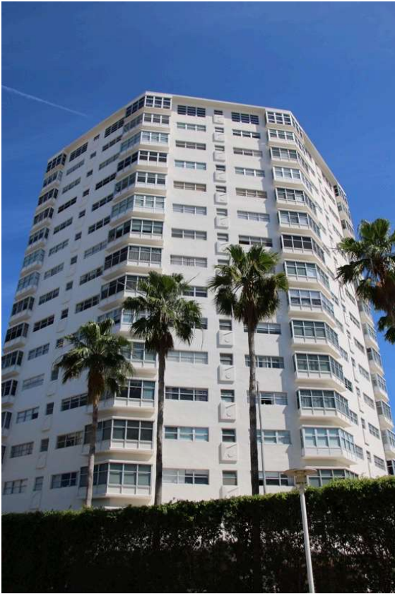
TOP LEFT: OCTAGON TOWERS ( ACROSS 19TH STREET)
