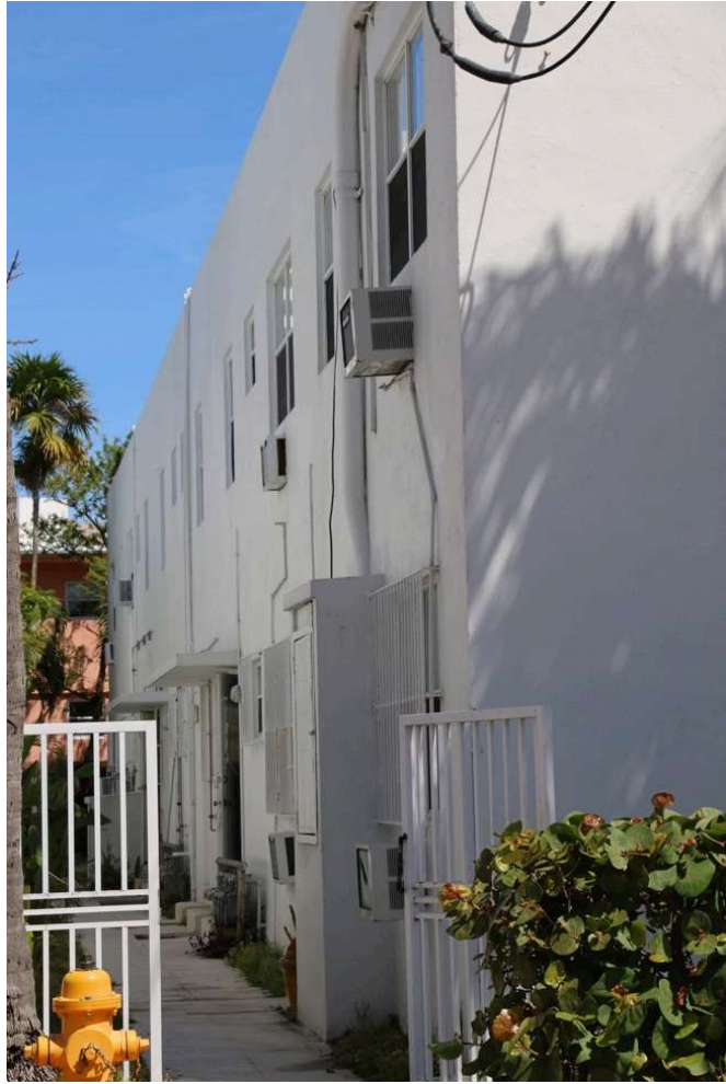
TOP LEFT PHOTO: 2018 PHOTOGRAPH OF NORTHERN ELEVATION (7)
