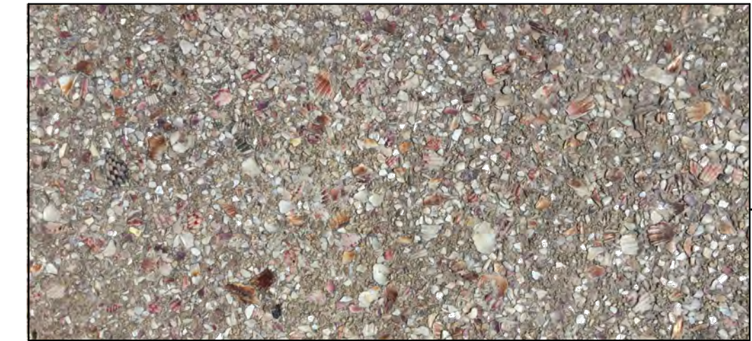
24"x24" CONCRETE PAVERS WITH CRUSHED SHELLS INSIDE PROPERTY. MIAMI BEACH STANDARD RED CONCRETE ON SIDE WALK
