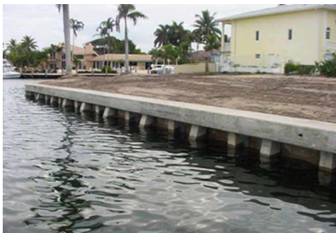
Figure 1. Seawall constructed with traditional flat concrete seawall panels
