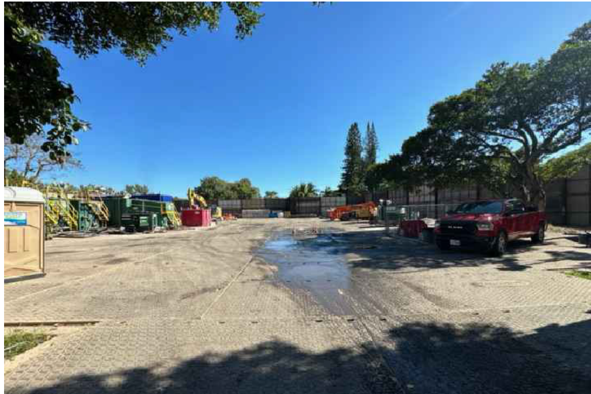
13. INSIDE FPL STAGING AREA
