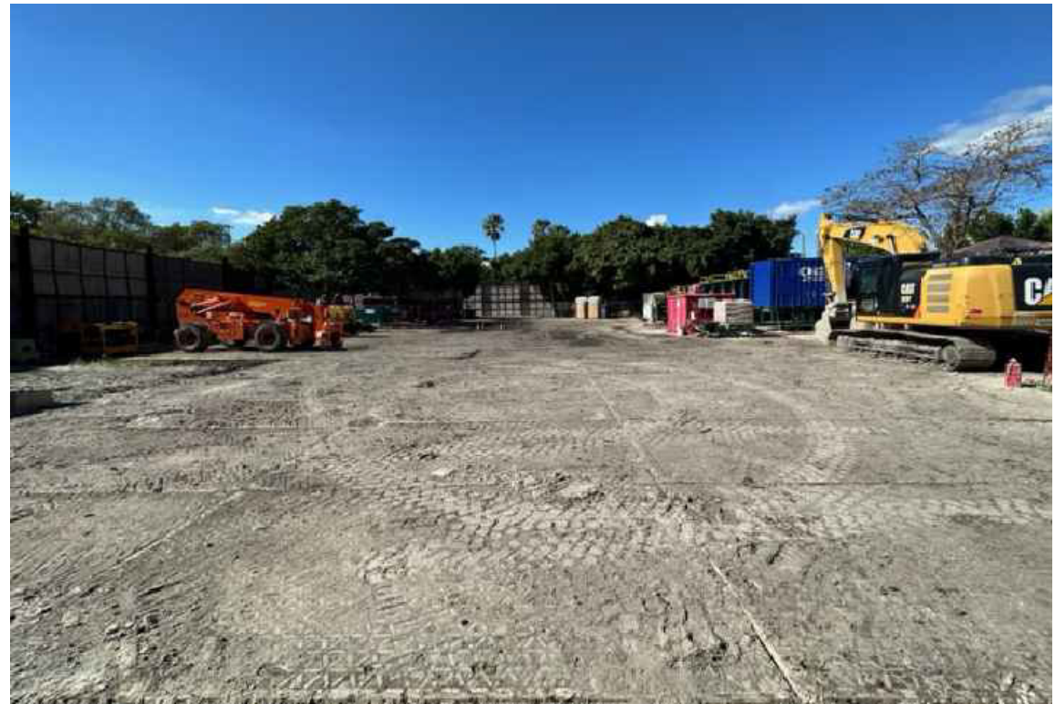
15. INSIDE FPL STAGING AREA FACING MICHIGAN AVENUE
